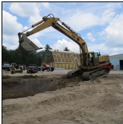
Site prep at town garage site
