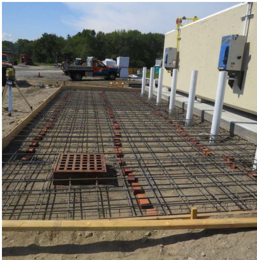
Town Garage Construction
