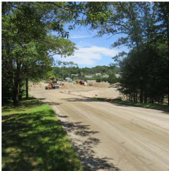
Site Preparation at the new DPW Garage
