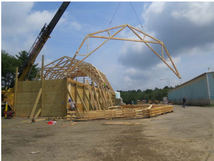
Salt Shed Construction
