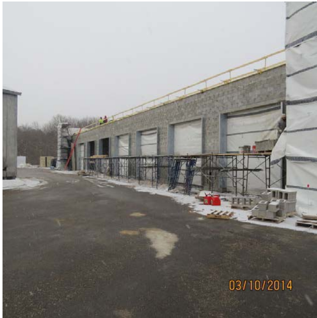
Ongoing construction at the DPW Garage
