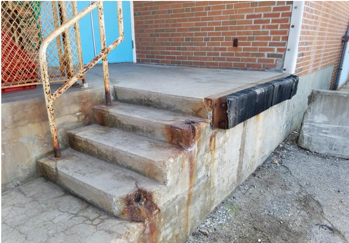
Showing deteriorated concrete steps, lack of handrail and areas needing paint
