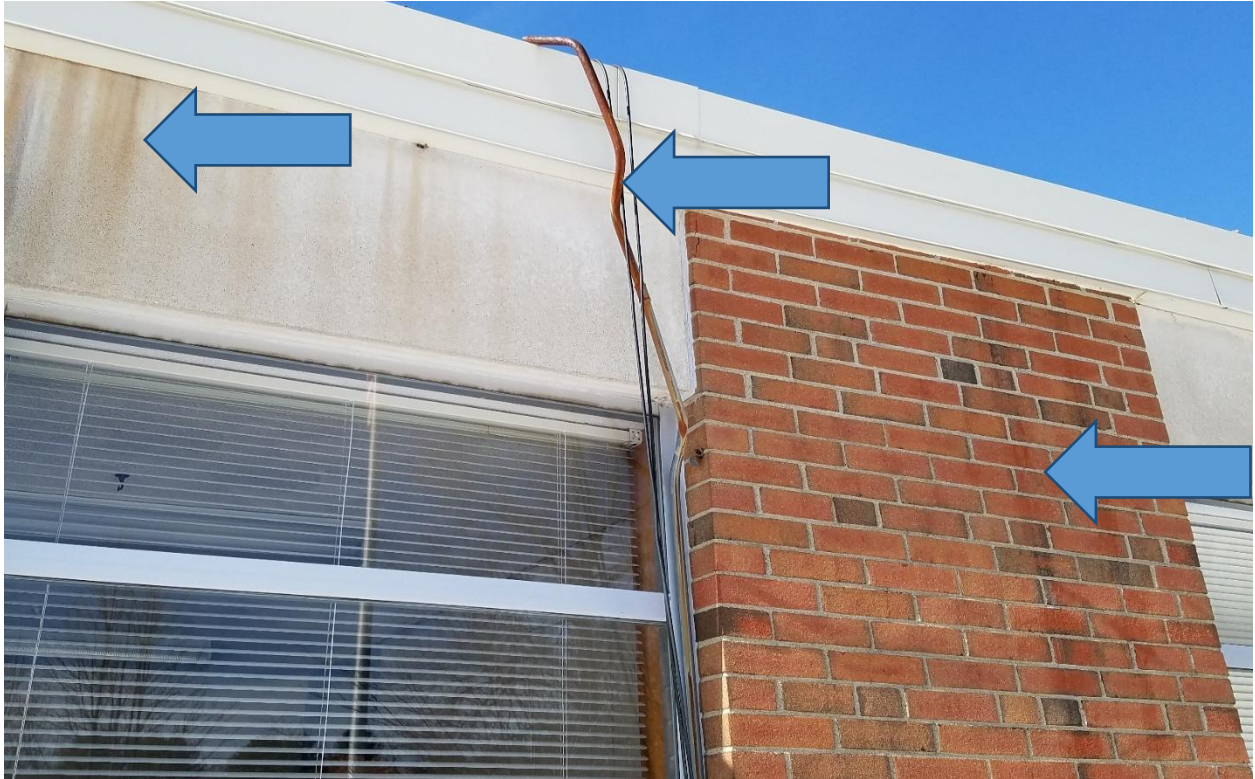
Showing stains from water infiltration from above / unsecured electrical conduits and moist brick
