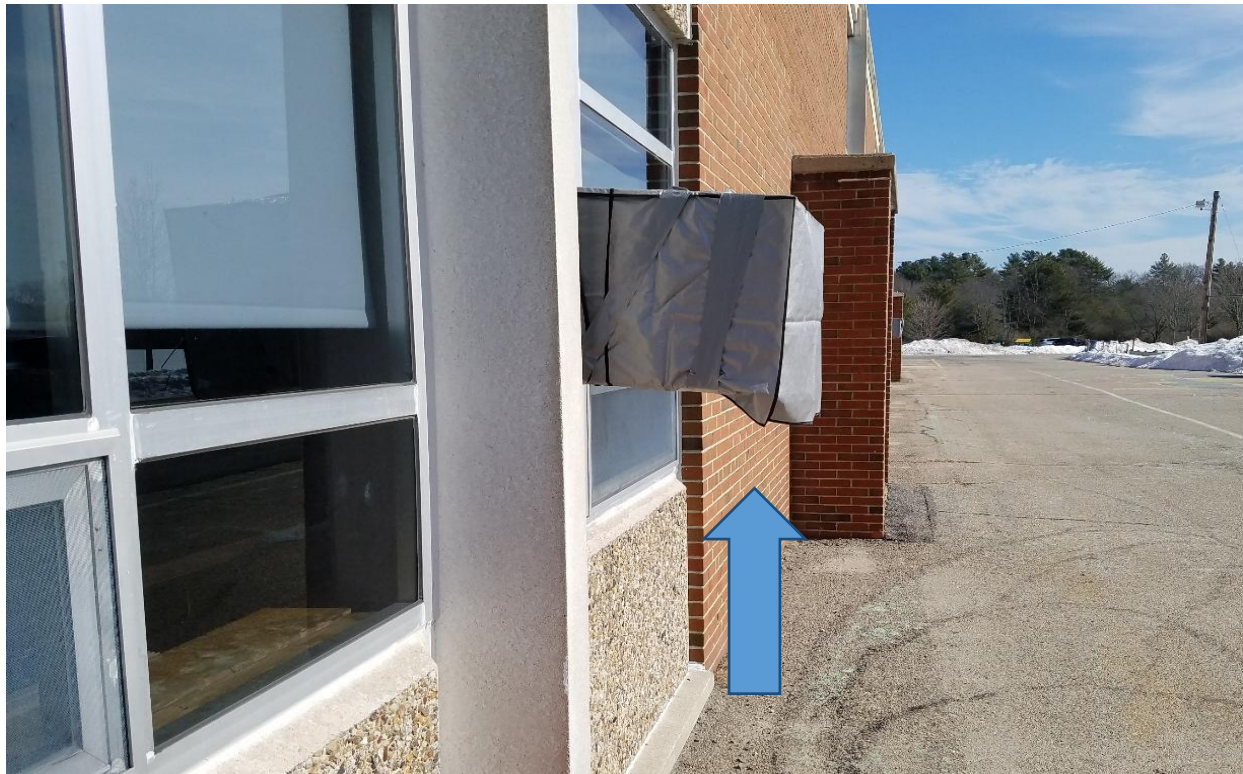
Potential hazard of protruding air-conditioner along walkway
