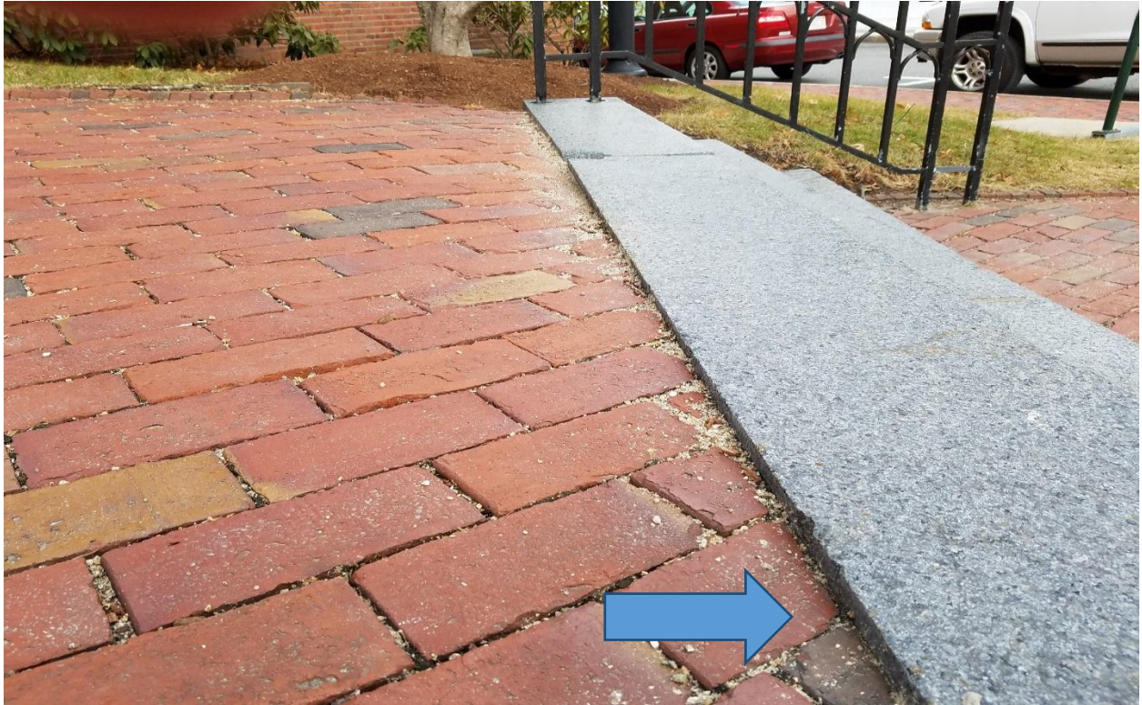
SHOWING LIP AT GRANITE TOP TREAD AND BRICK SETTLEMENT
