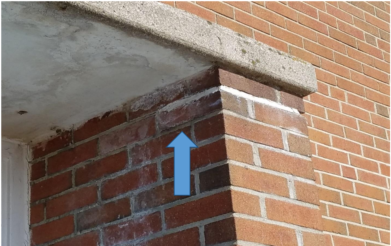
Another typical example of porous concrete entry cap that has caused brick deterioration
