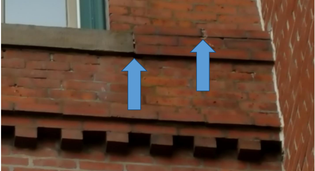
OPEN JOINTS IN BRICK/LIMESTONE
