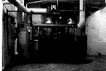
Boilers and water heater with flues
