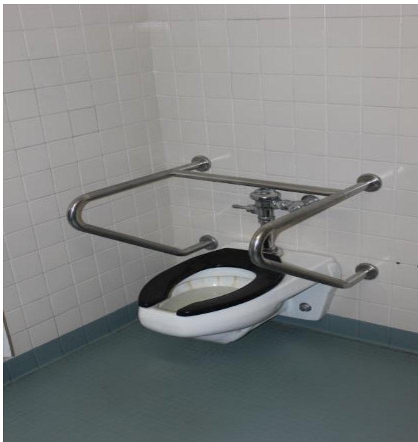
Gang bathroom retrofit for ADA compliance. Removed an adjoining toilet and installed handrail bars
