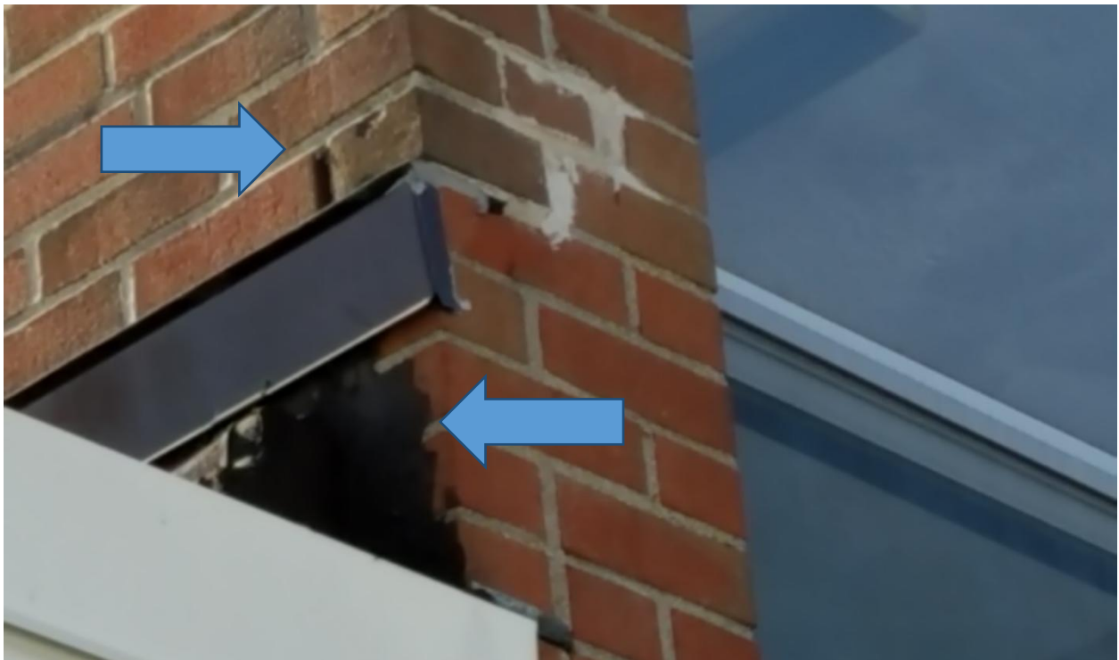
Poor roof flashing transition and open brick joints needing repair ( north elevation )
