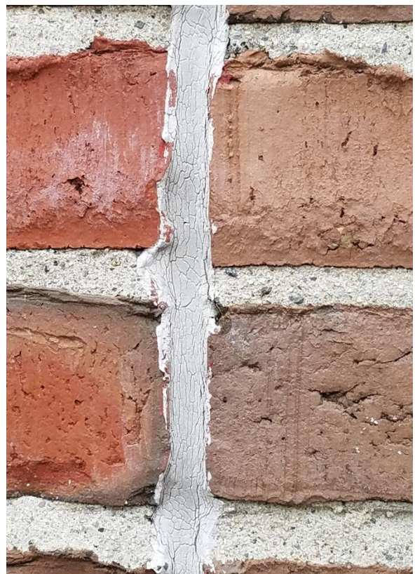
MASONRY CONTROL JOINT TO BE REDONE
