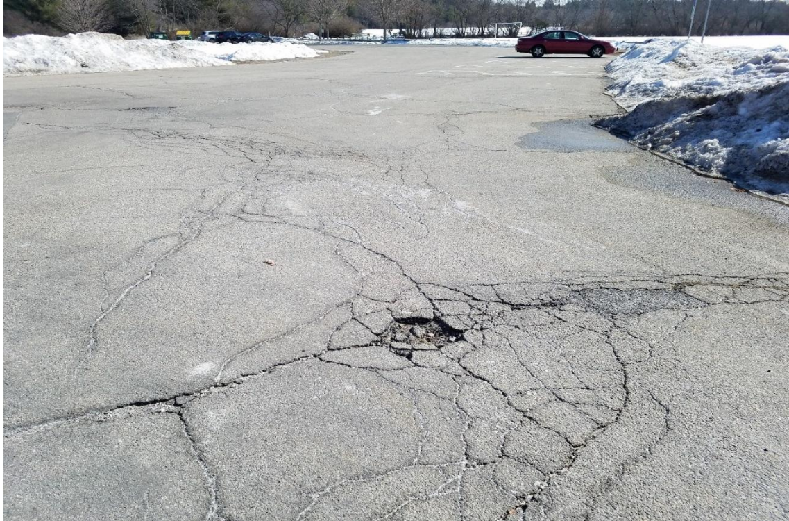
Showing deteriorated pavement and pothole at rear driveway area
