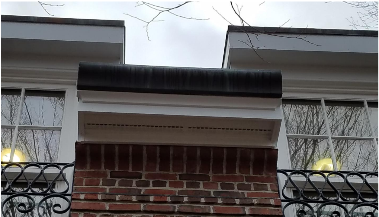
GUTTER WITH NO APPARENT DOWNSPOUT (EAST ELEVATION)
