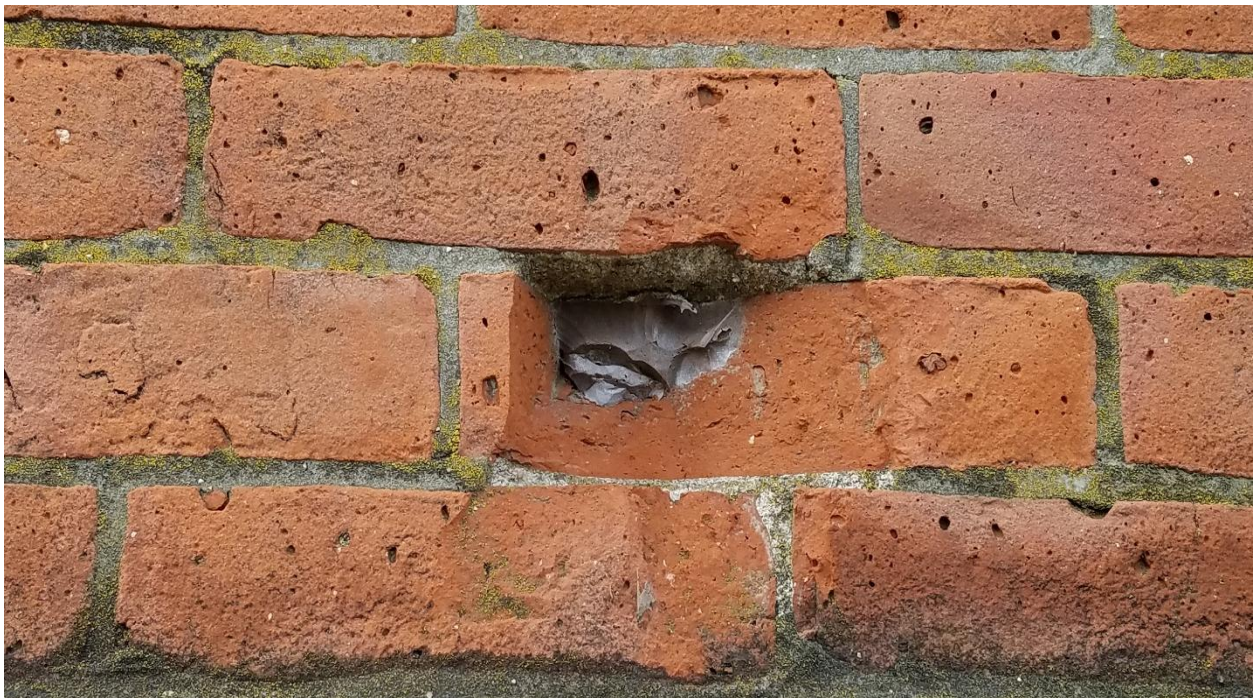
TYPICAL EXAMPLE OF SPALLED BRICK NEEDING REPLACEMENT and GROWTH ON BRICKS & MORTAR
