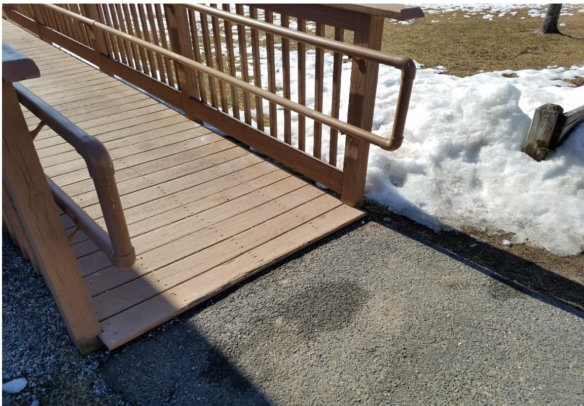
Showing tripping hazard lip at edge of ramp and non-compliant rail system at After School Center
