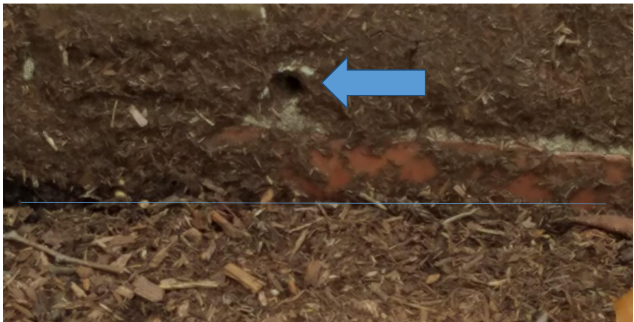
SHOWING TYPICAL CLOGGED WEEP HOLES DUE TO MULCH
