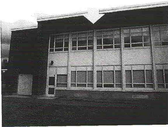
Roof-Wall Intersection Air Sealing – there are exterior vent plugs in place; this construction directs outdoor air at the weak seal (see top right picture) at the roof-wall intersection, leading to excessive infiltration/ exfiltration.
