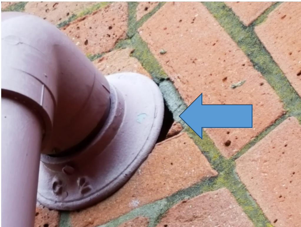
GAPS AROUND SPRINKLER DRAIN NEEDING SEALANTS
