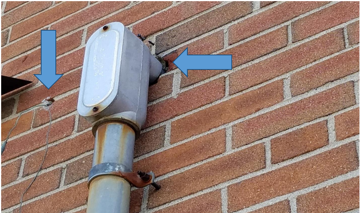
Example of brick penetrations needing sealant ( west elevation )
