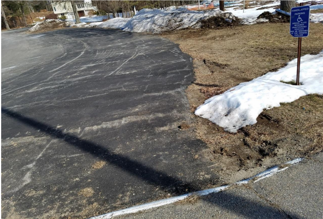
Showing lack of pavement markings and excessive slope at accessible parking space
