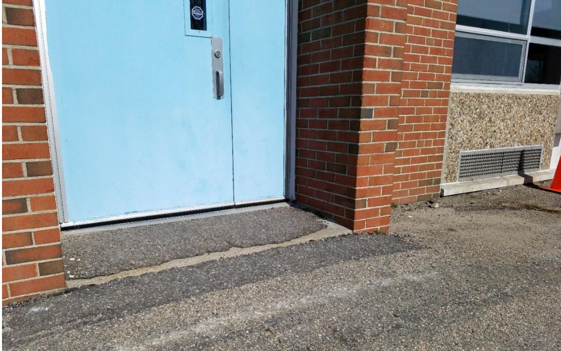
Another example of no 5' level landing at egress doors, currently poorly patched with bituminous
