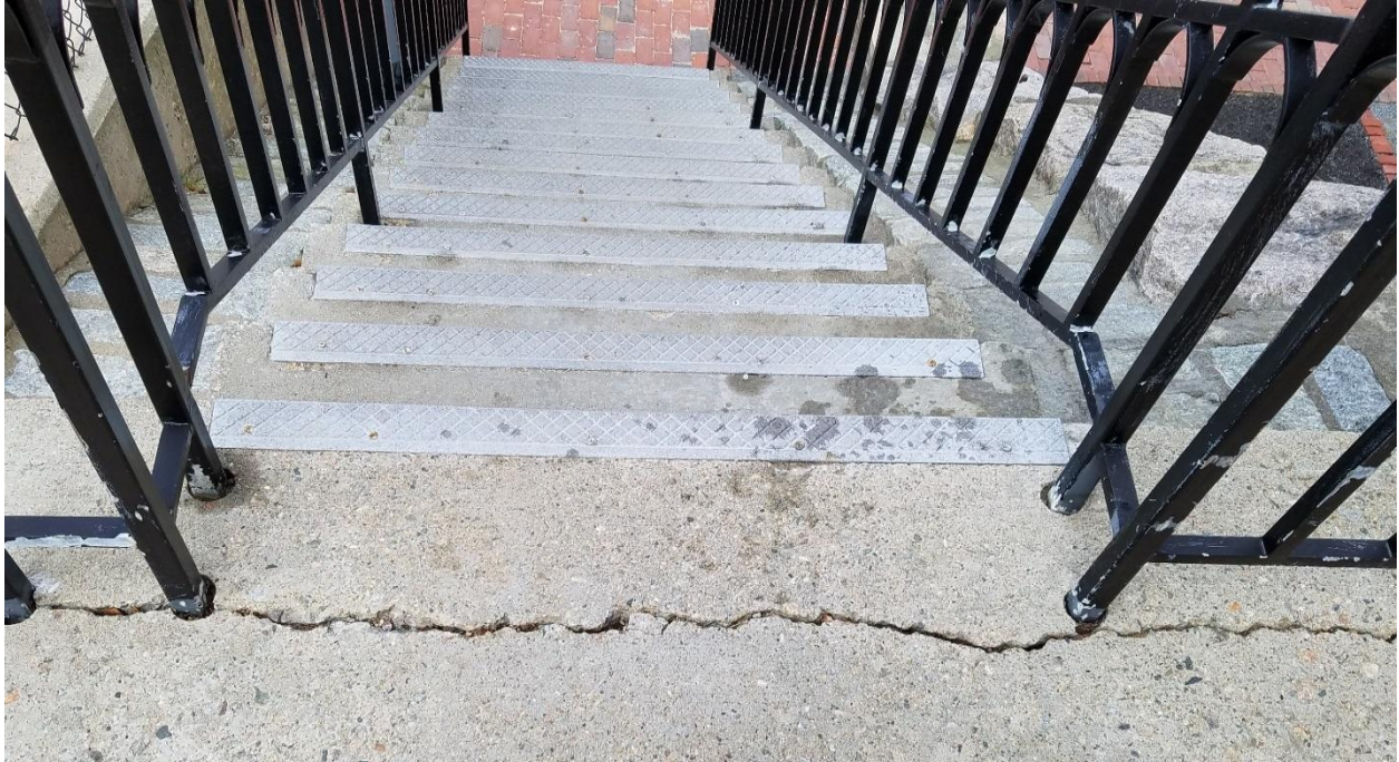
CONCRETE STAIRS & HANDRAILS FROM LOWER (REAR) LEVEL TO MAIN STREET ENTRANCE LEVEL ( Note crack at top tread )
