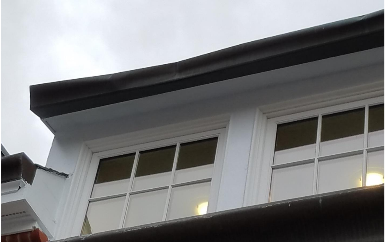
EXAMPLE OF DAMAGED GUTTERS (WEST ELEVATION)
