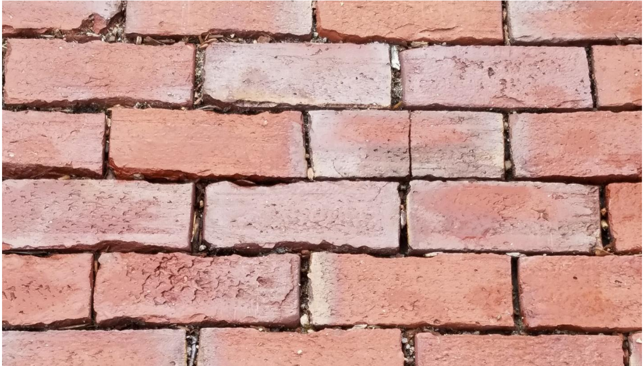
TYPICAL OPEN JOINTS OF BRICK WALKWAYS NEEDING SAND INFILL
