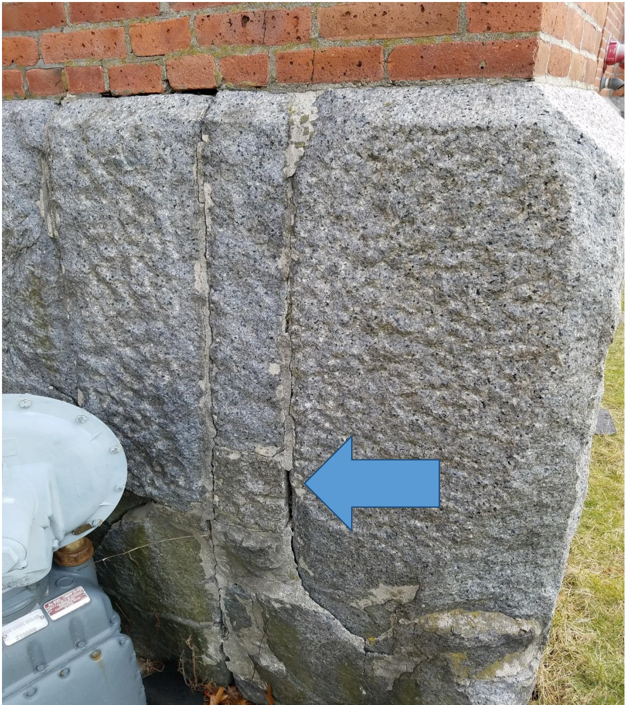
TYPICAL CRACKS IN GRANITE FOUNDATION CAP STONES
