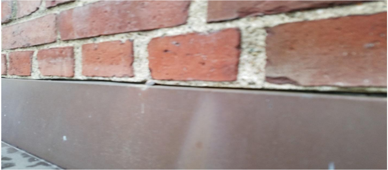
OPEN FLASHING JOINT AT REAR ELEVATION ABOVE STANDING SEAM ROOF
