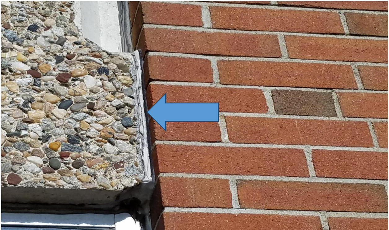
Typical joint between precast and brick needing to be re-sealed
