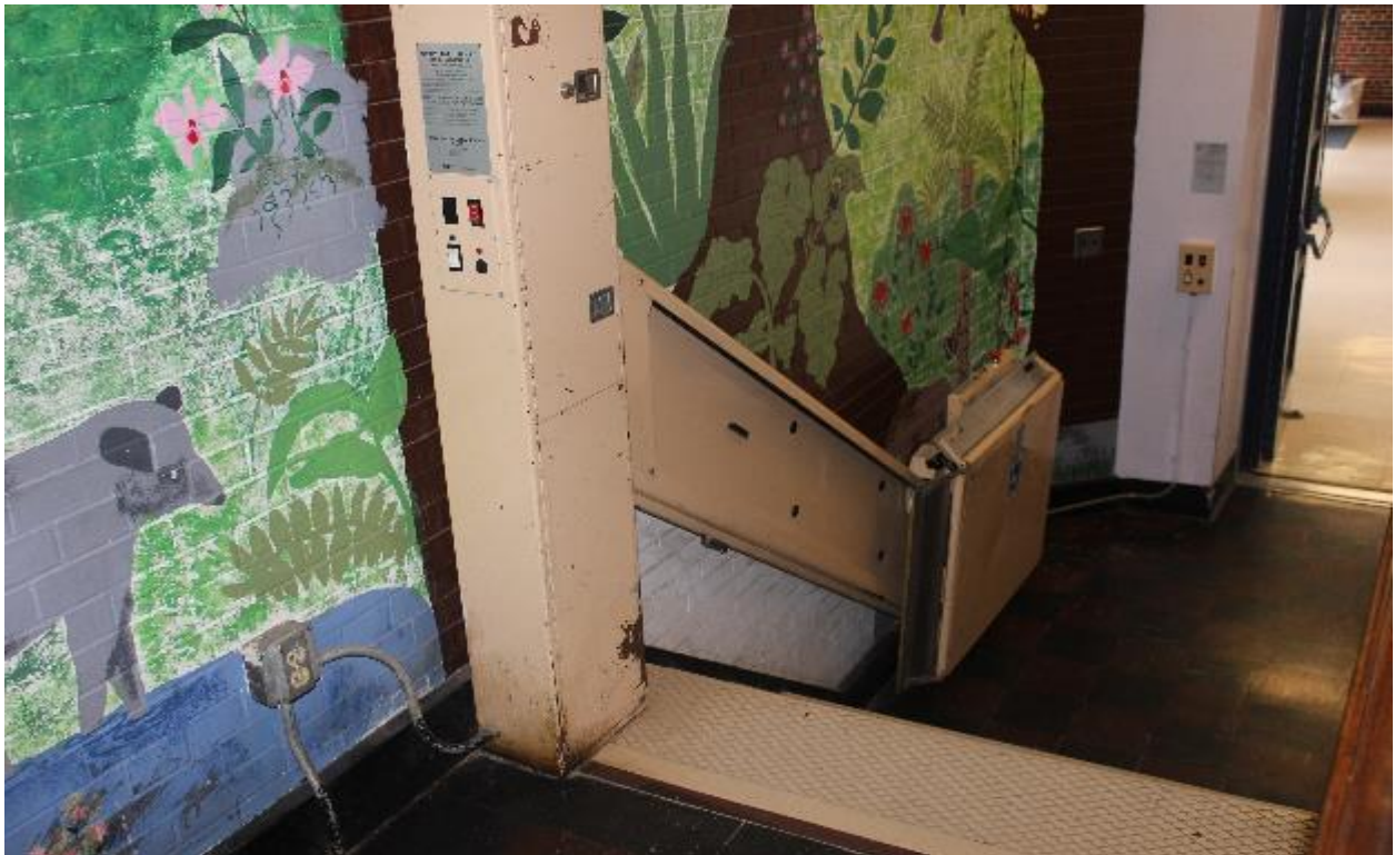
Handicap accessible lift in stair (No longer allowed by code) Note no elevator to second floor.
