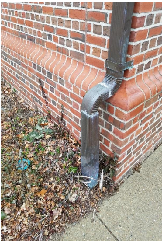
DAMAGED DOWNSPOUT
