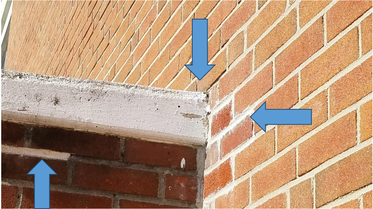
Sloped concrete entry cap with no protective membrane and no flashing to vertical brick surface – also signs of brick deterioration and previous repairs
