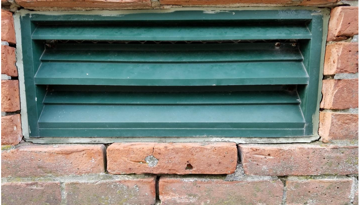
OPEN JOINTS IN BRICK AROUND OPENINGS CREATED DURING 1998 RENOVATIONS
