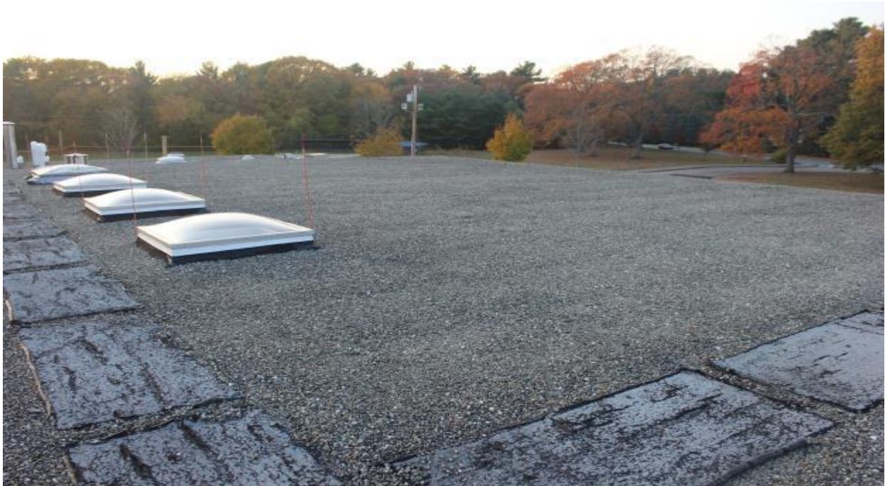
BUR roof Thinning stone ballast, walk pad failing, curb flashing is separating from vertical rise.
