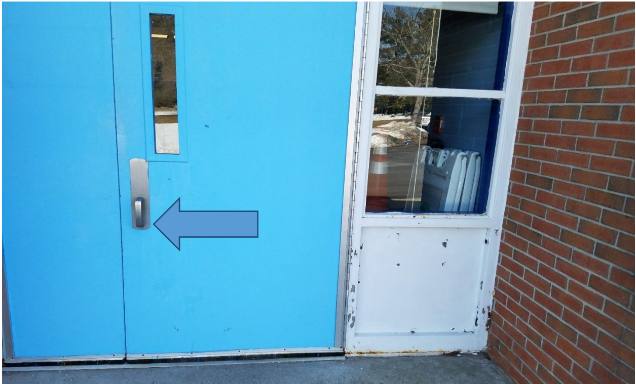
Typical entry showing non-compliant door latching hardware and hollow metal frames needing paint
