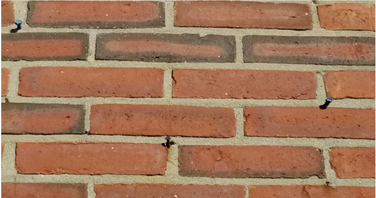
Example of old fasteners that should be removed and patched with mortar or caulking
