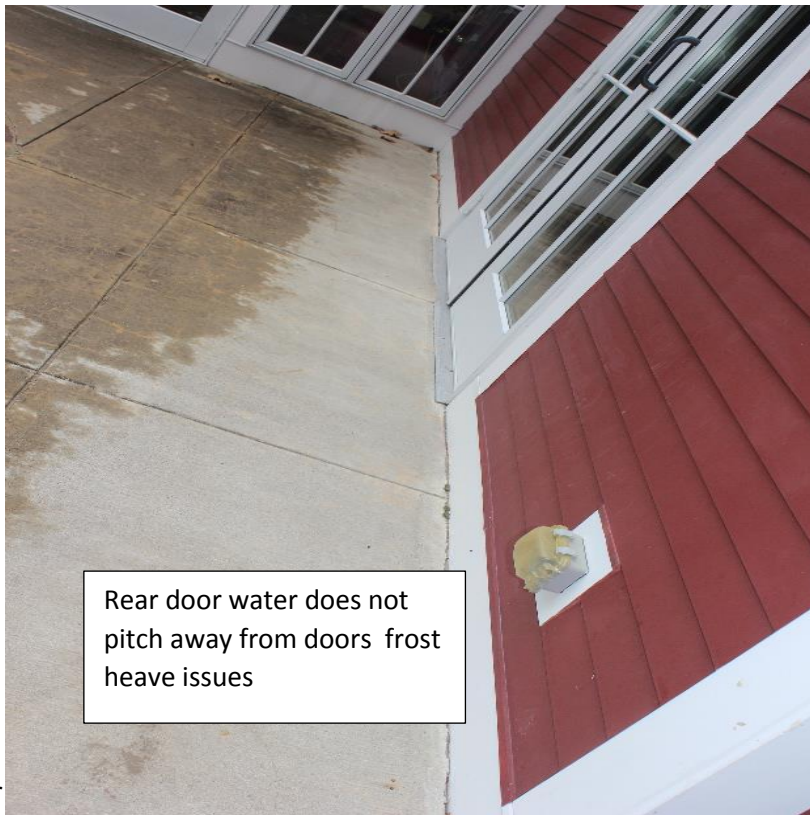
Poor drainage has led to frost heaving and door failure to open. All locations
