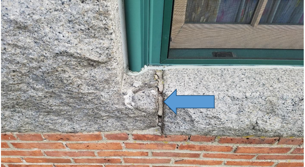
SHOWING REPOINTING NEEDED AT GRANITE SILLS
