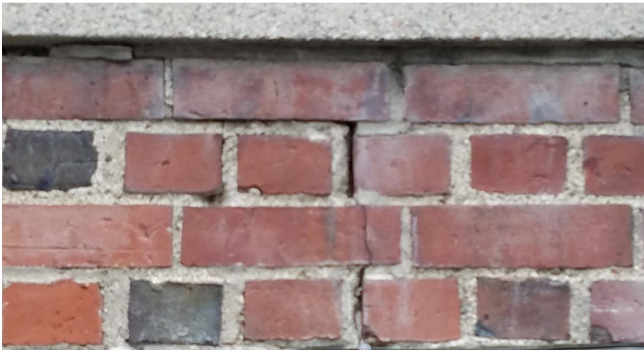
OPEN BRICK JOINTS TO BE REPOINTED (REAR ELEVATION)
