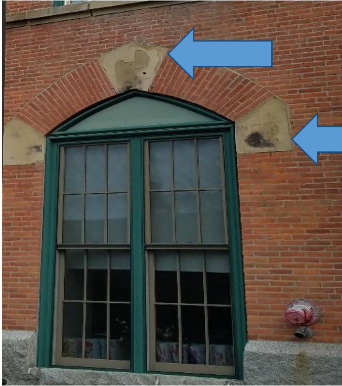
TYPICAL DETERIORATED LIMESTONE KEYS
