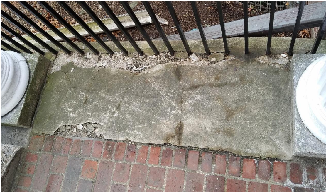
DETERIORATED EDGES OF ORIGINAL ENTRY PLATFORM (NORTH ELEVATION)
