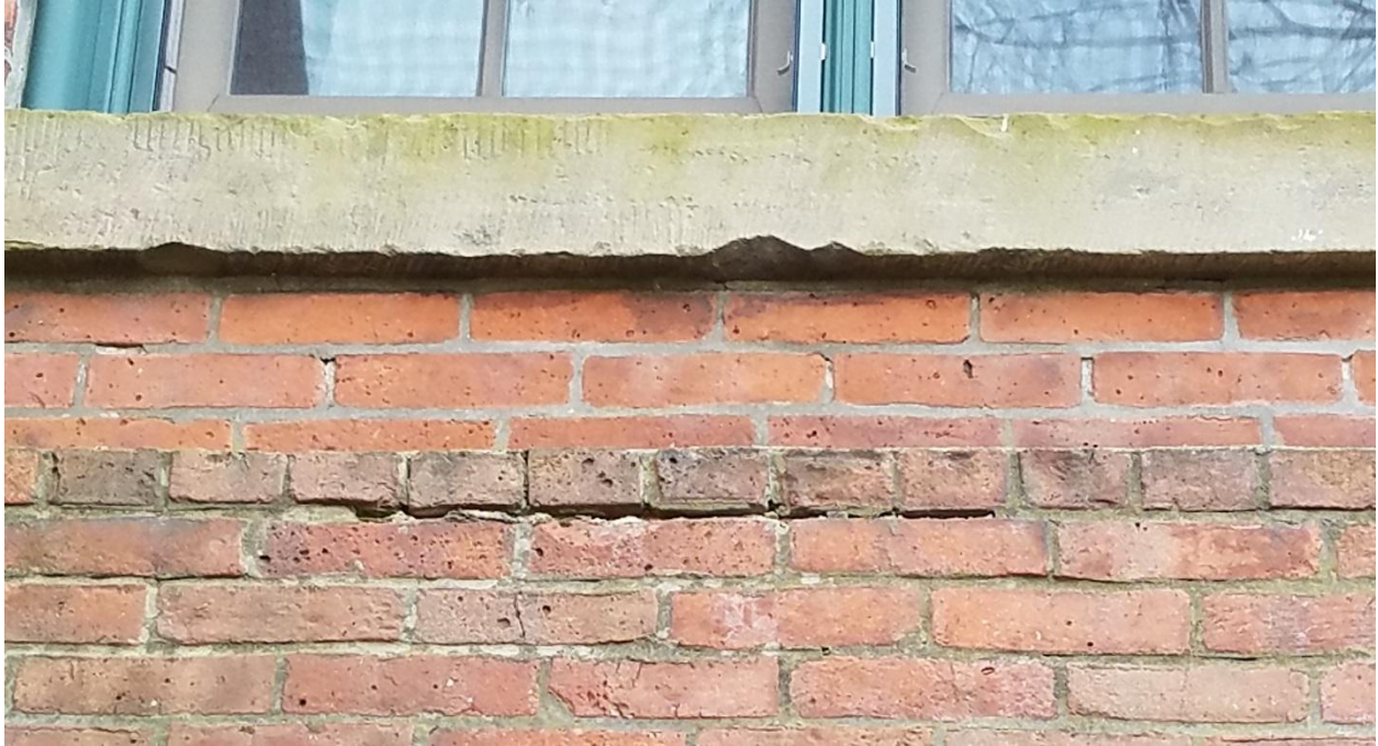
TYPICAL EXAMPLE OF DETERIORATED LIMESTONE SILL and OPEN JOINTS AT INTERMEDIATE WATER TABLE BRICK
