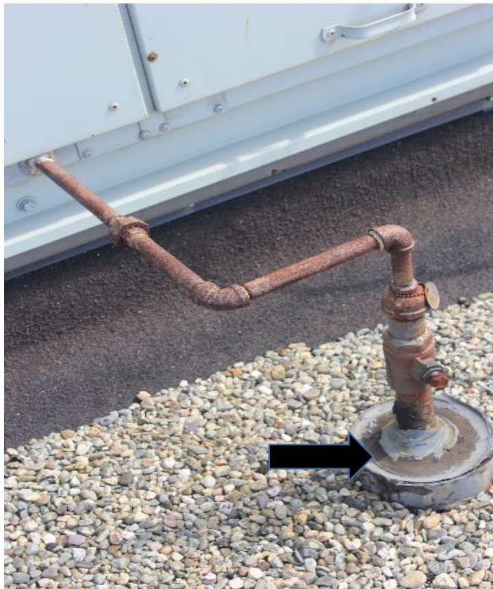
BUR flashing at HVAC and poor pitch pocket
