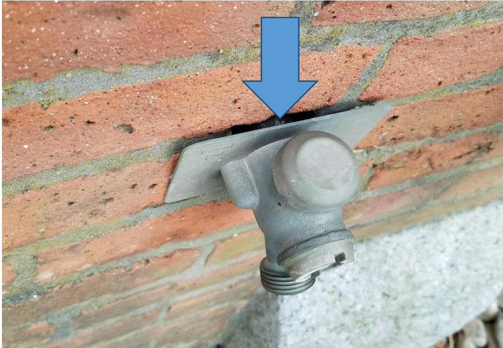
GAPS AROUND EXTERIOR HOSE BIBS NEEDING SEALANTS
