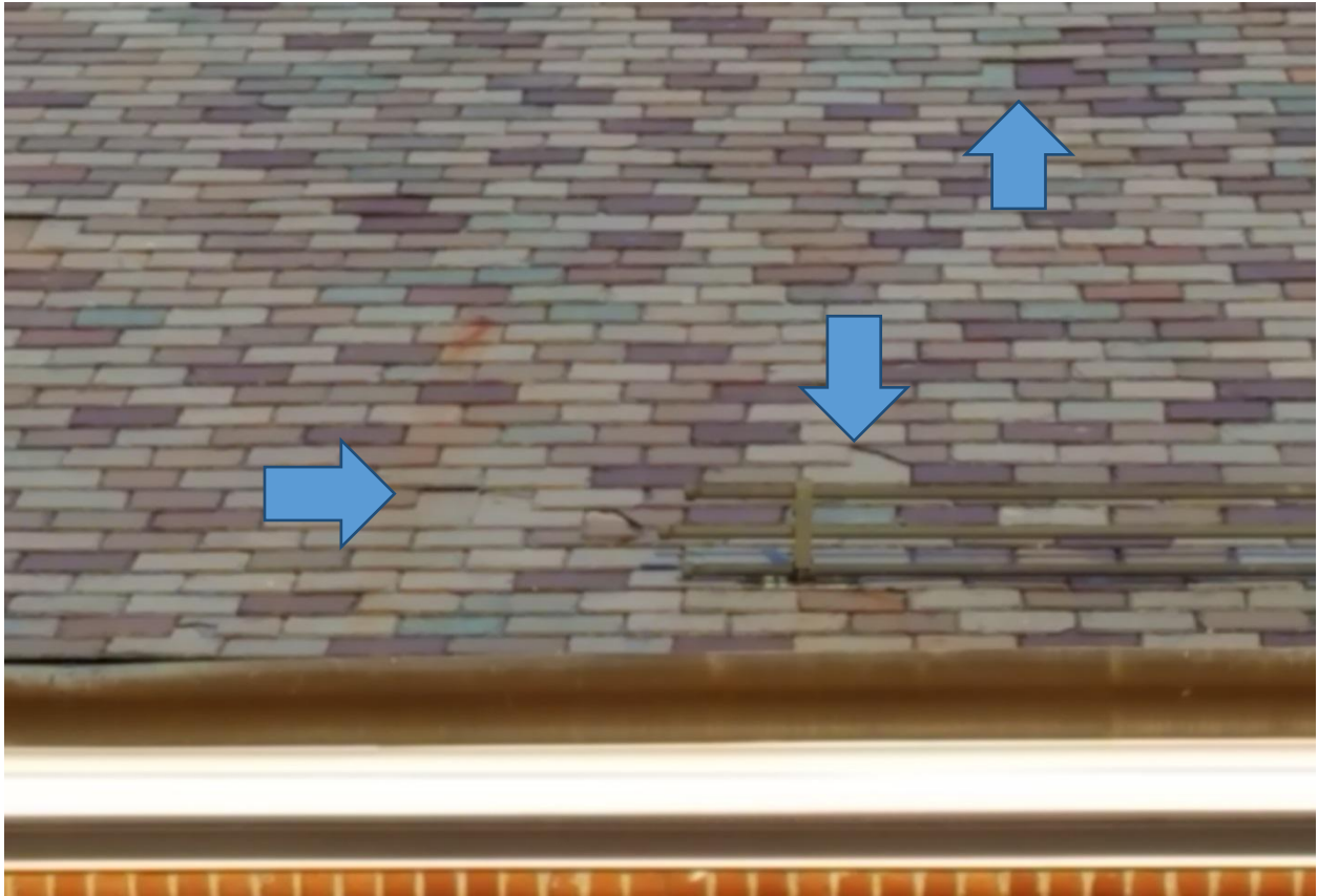
WEST-FACING SLATE ROOF SHOWING MISSING SLATES
