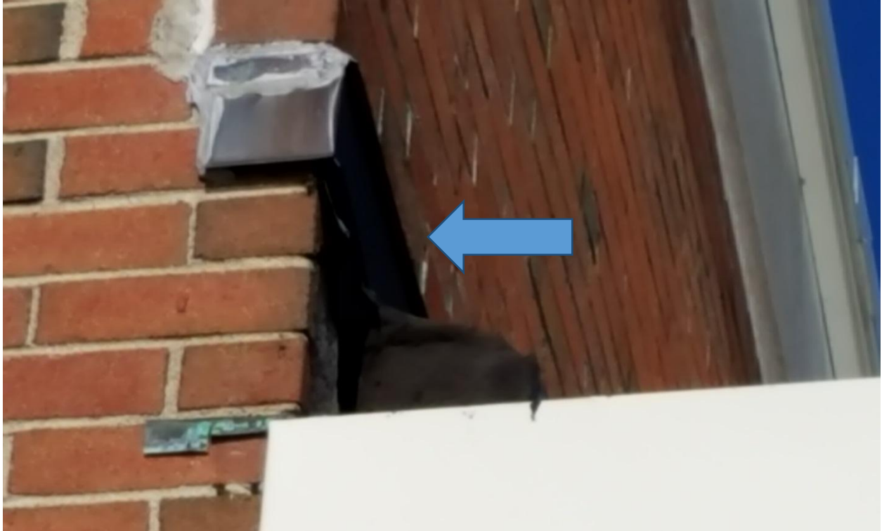
Another example of poor flashing transtion ( South elevation )
