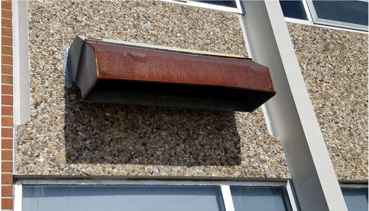
Typical rusted condition of second floor UV louver hood needing replacement
