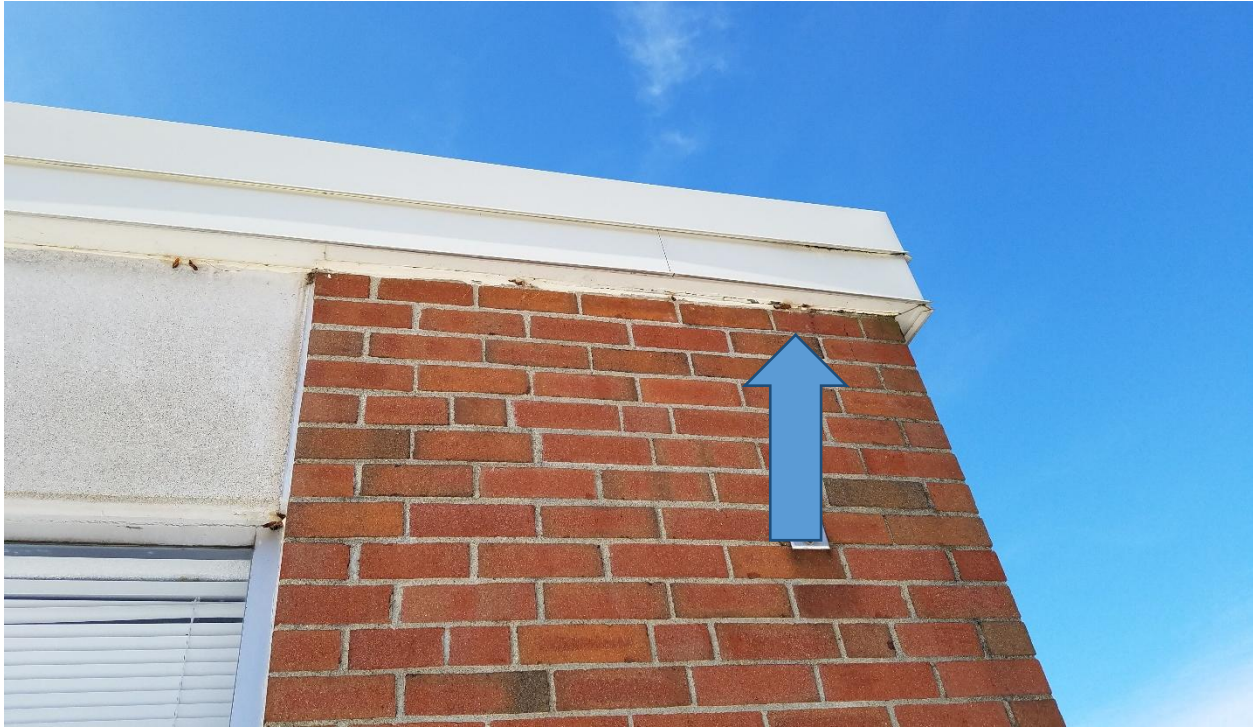
Typical horizontal joint needing to be resealed
