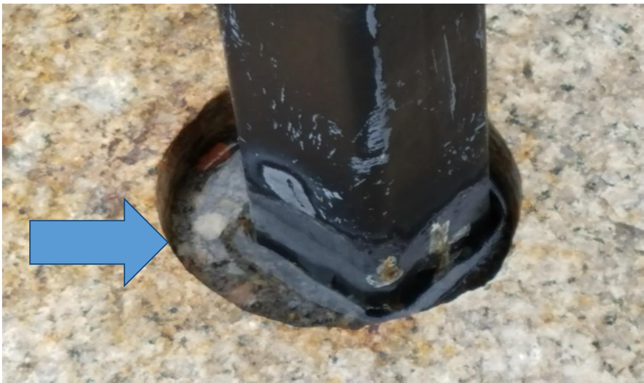
GAPS AROUND GUARDRAIL POSTS COLLECTING WATER & ICE
