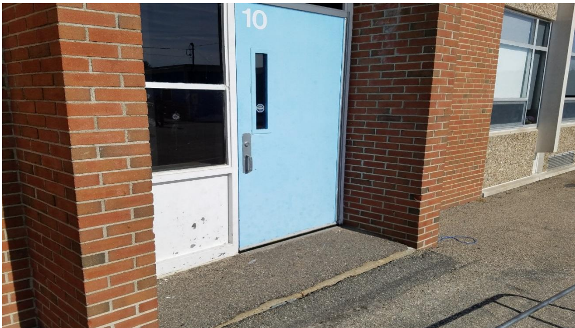
Showing lack of 5' level landing at egress door and HM frames needing paint
