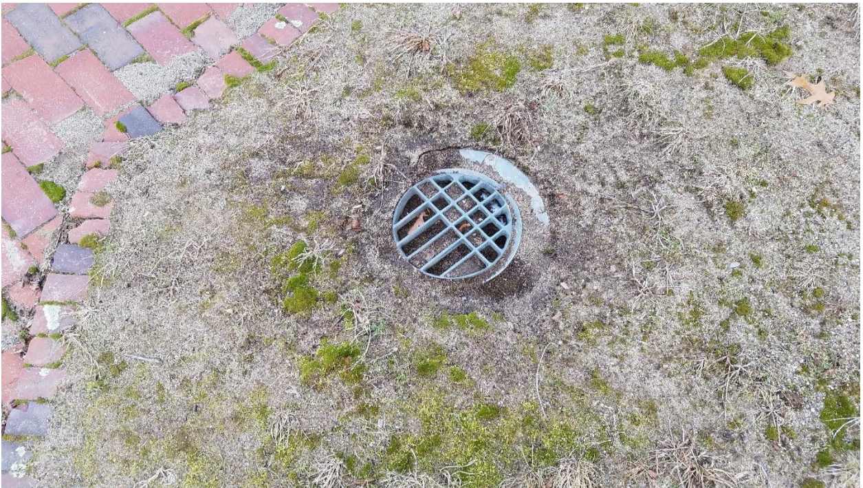
TYPICAL LANDSCAPING LIGHTS FILLED WITH DEBRIS
