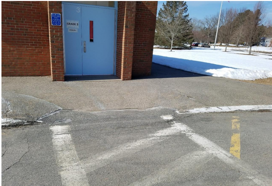
Poorly constructed curb cut and worn pavement markings
