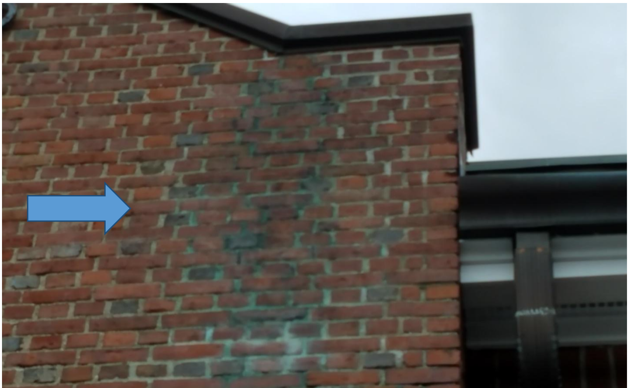
POSSIBLE LEAK AT PARAPET COPING CAUSING INFILTRATION INTO WALL & EFFLORESCENCE
