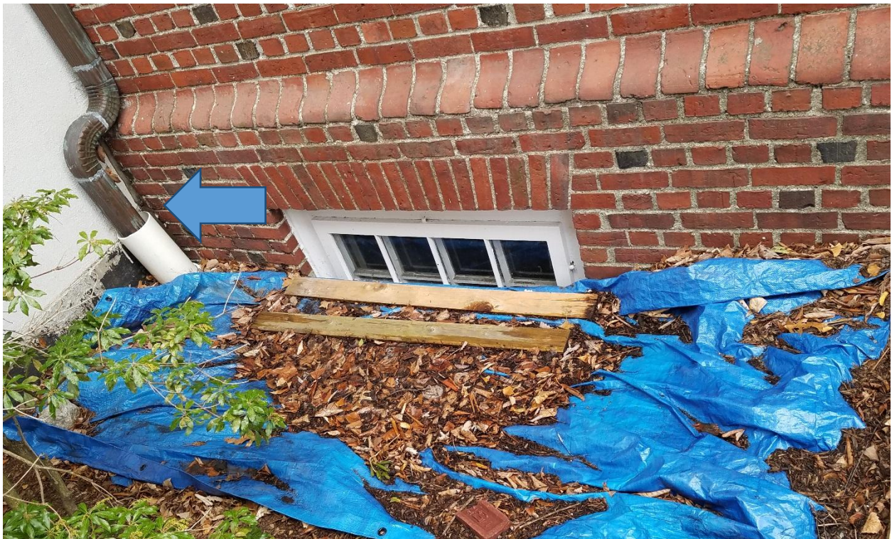
AREA WELL WITH TEMPORARY FIX and NOTE OPEN DOWNSPOUT JOINT (ARROW)
