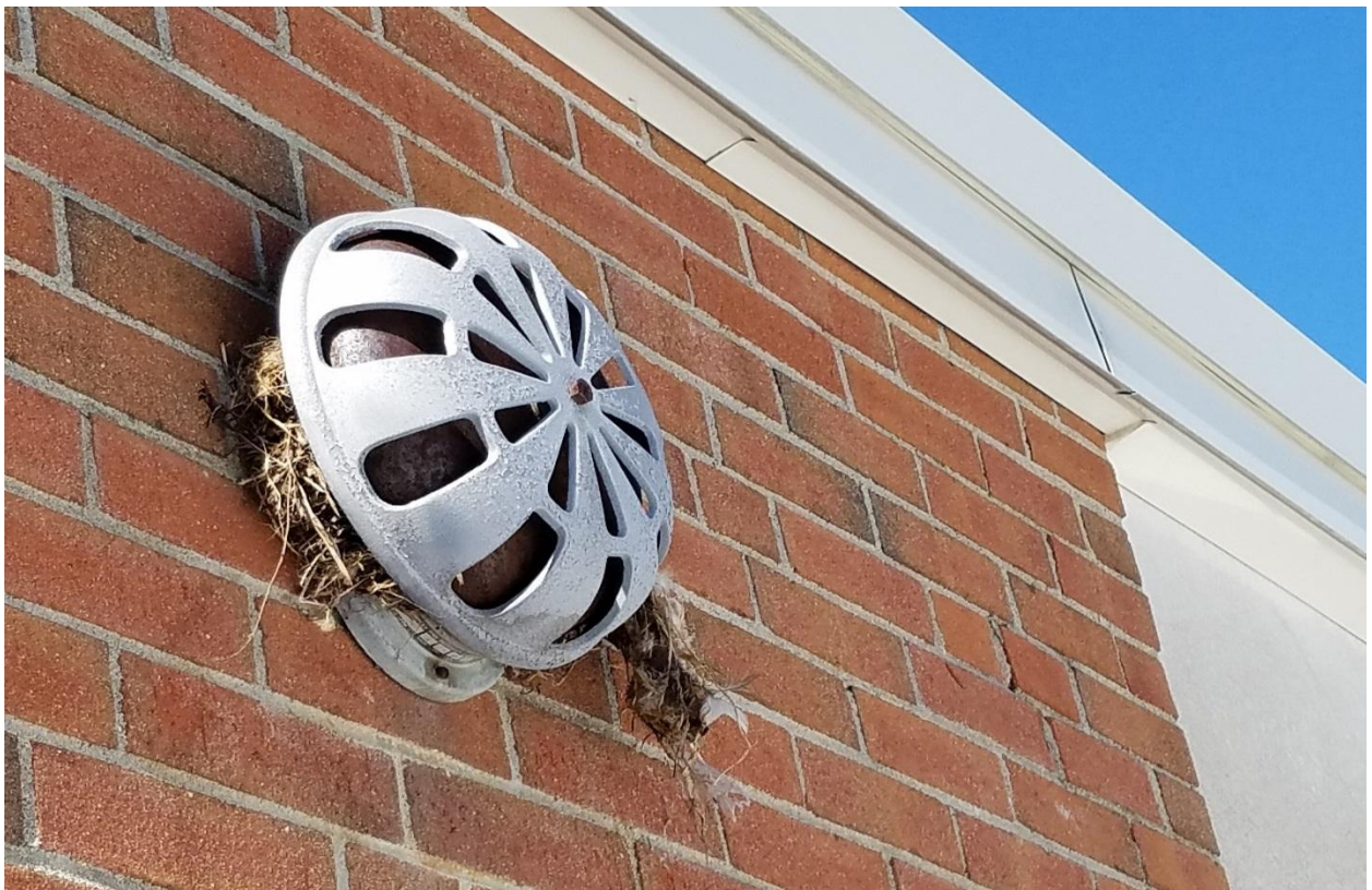
Example of abandoned exterior fixtures that should be capped or removed and infilled with brick
