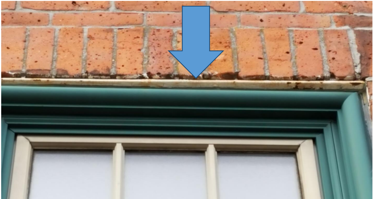
TYPICAL STEEL LINTEL NEEDING SCRAPE & PAINT
