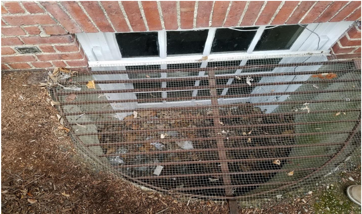
SHOWING TYPICAL AREA WELL NEEDING DEBRIS REMOVED
