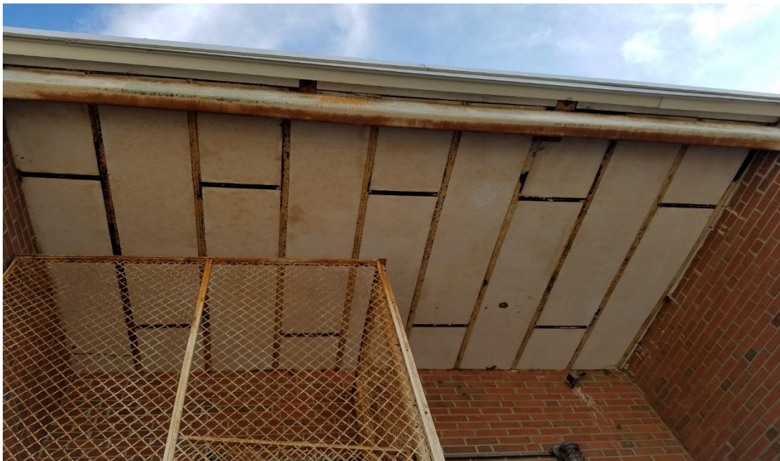
Rusted metal components at covered truck dock ( West )
