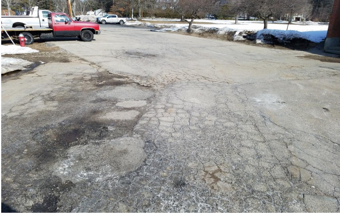
Showing poor condition of paving on west side and routine parking on lawn areas
