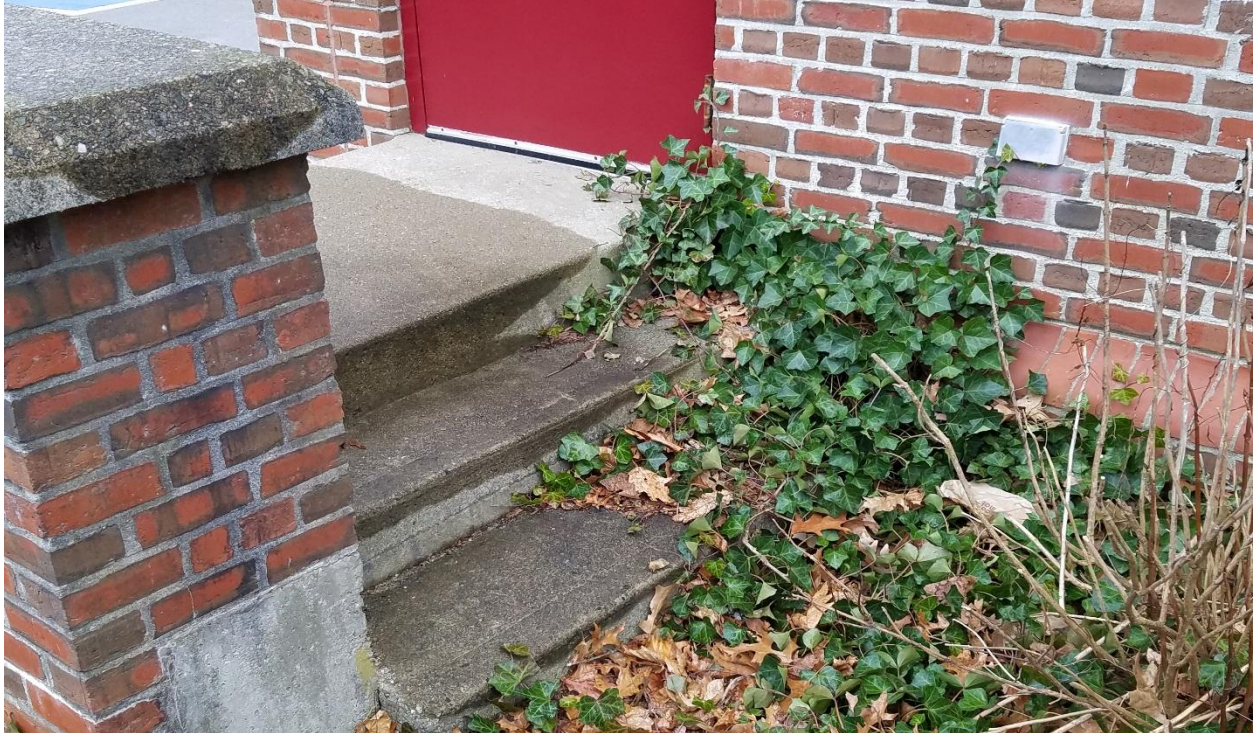
3-RISER STEPS WITH NO HANDRAILS and OVERGROWN WITH VEGETATION (EAST ELEVATION)
