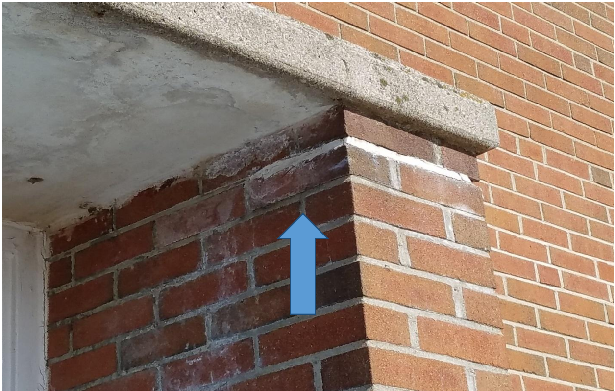
Showing water penetration through concrete entry cap deteriorating brick (efflorescence shown )
