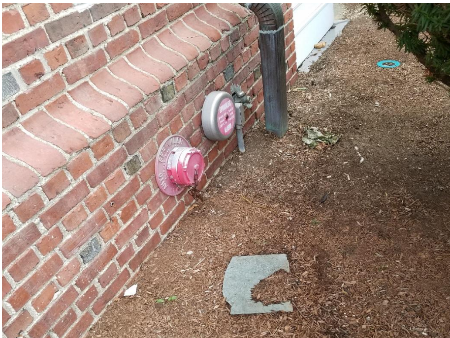
SHOWING DEMINISHED ACCESS TO FIRE DEPARTMENT CONNECTION (WEST) (NOTE FALLEN ROOF SLATE IN FOREGROUND)
