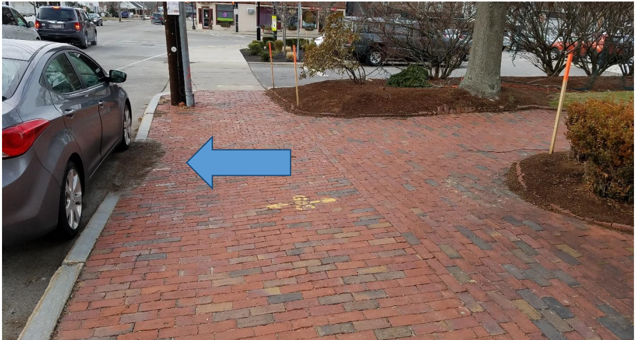
SHOWING MAIN STREET CURB CUT WITH NO DESIGNATION FOR ACCESSIBLE PARKING
