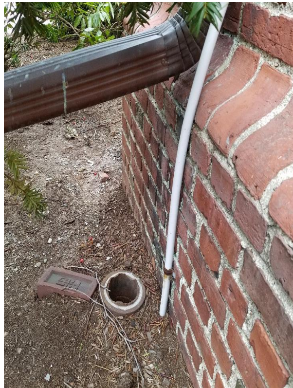
UNCONNECTED DOWNSPOUT
