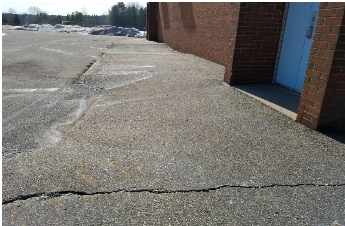
Egress door lacking 5' level landing before slope to curb cut, and deteriorated paved walkway
