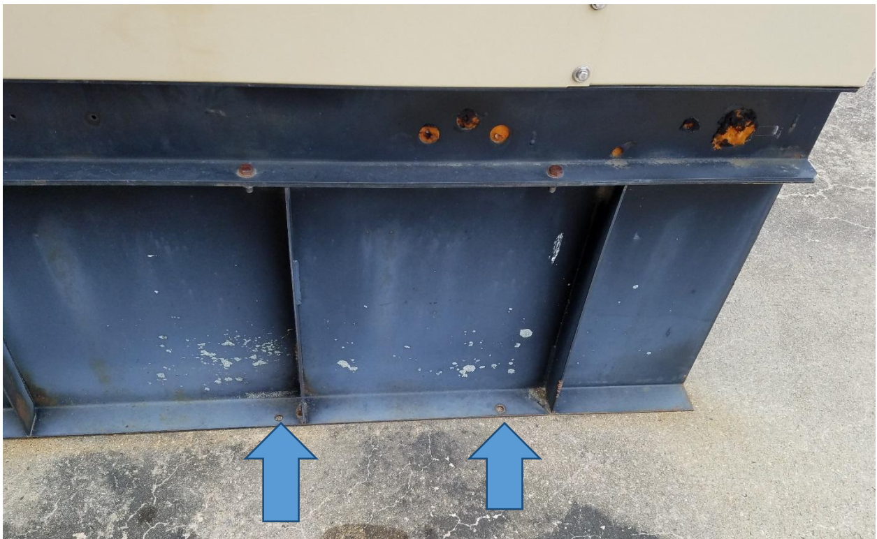
GENERATOR UNSECURED TO CONCRETE PAD
