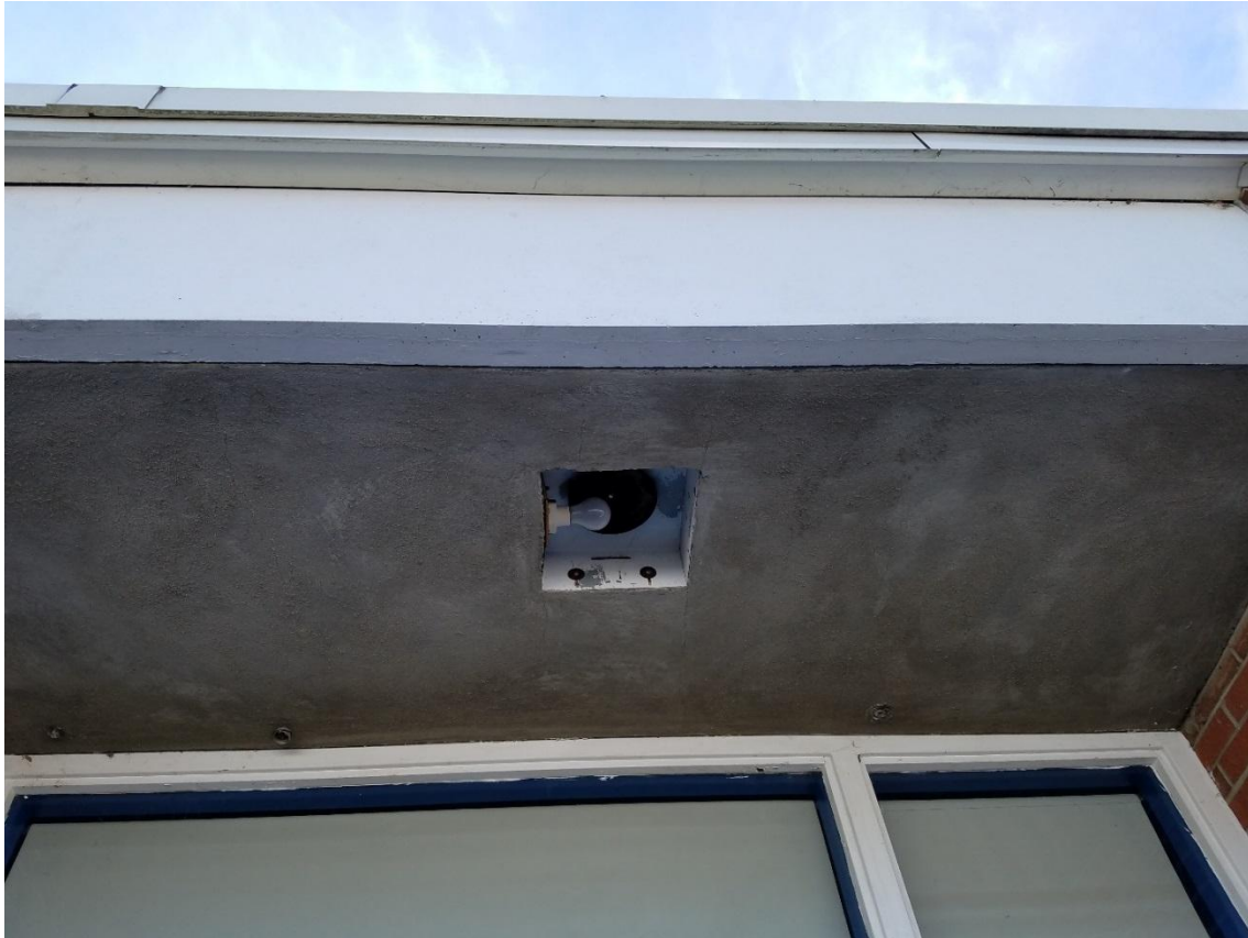
Outdated incandescent fixture and water-stained ceiling of covered entry
