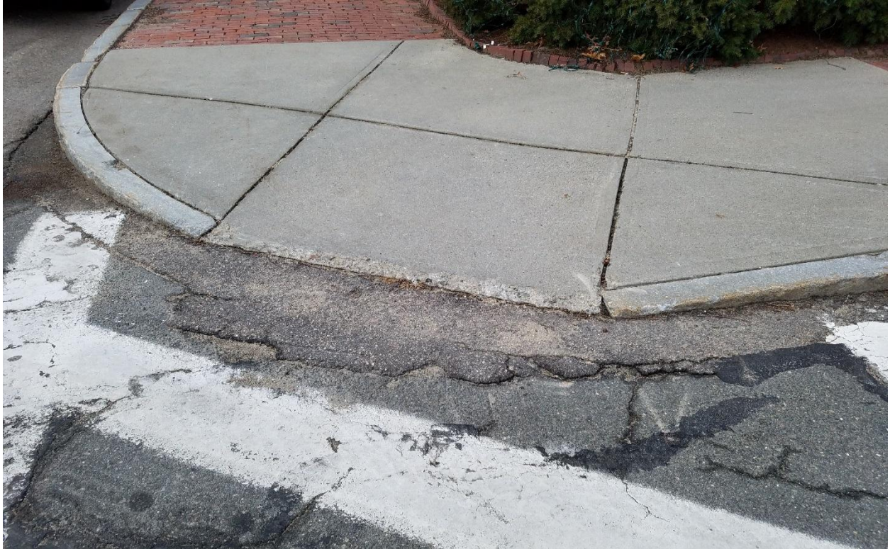
SHOWING POOR CONDITION OF CURB CUT AND PAVING AT JANES AVE CROSSWALK
