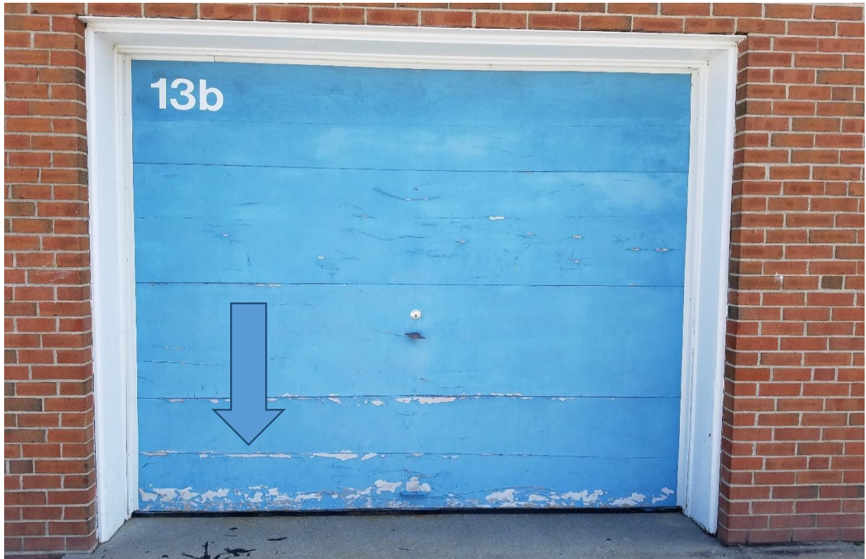
Showing delaminated veneer on garage doors
