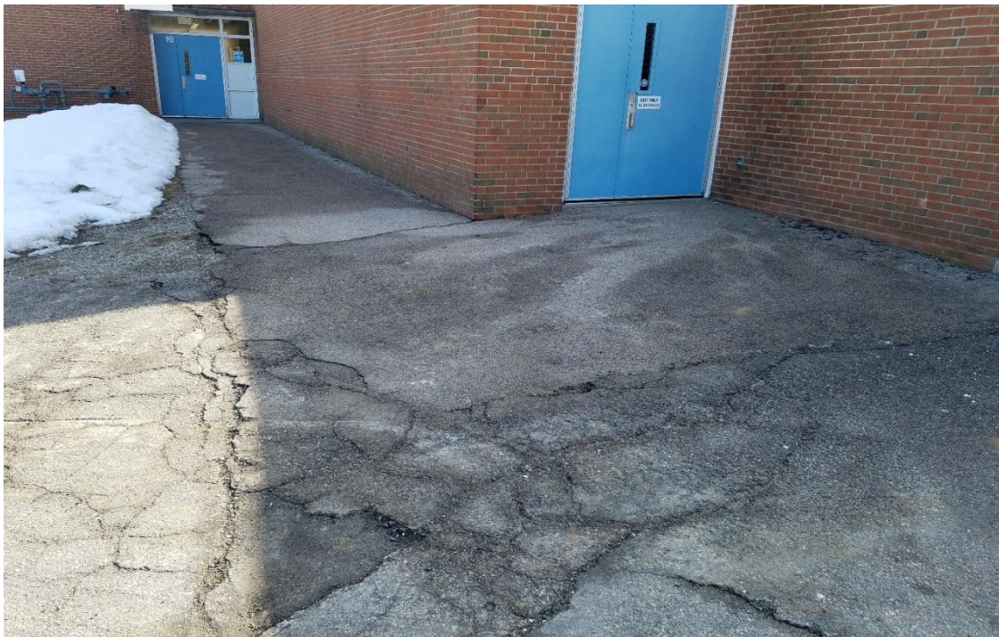
Deteriorated paving at egress path from exits
