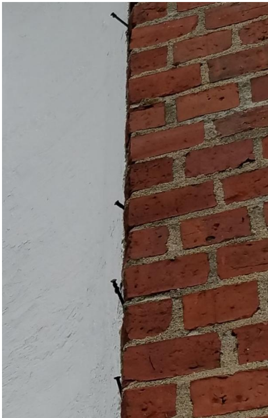
RUSTY OLD FASTENERS TO BE REMOVE
