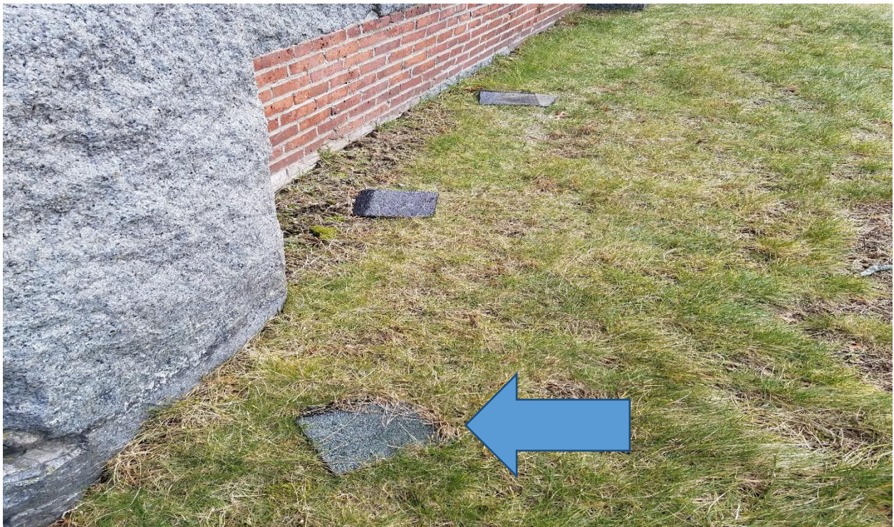
FALLEN ASPHALT SHINGLED SCATTERED AROUND BUILDING PERIMETER
