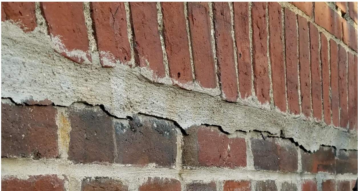
POORLY EXECUTED REPOINTING (WEST ELEVATION)
