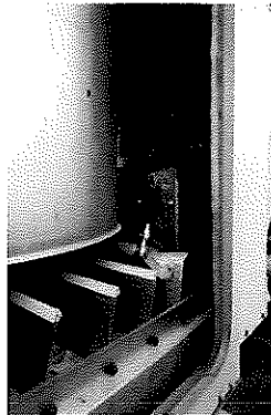
Internal return and economizer dampers and control
