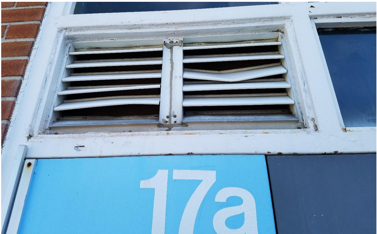
Example of mechanical louver needing repair/replacement
