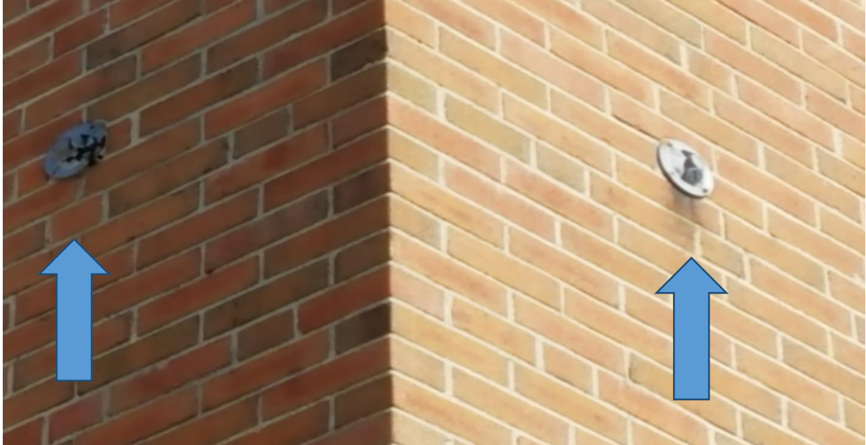
Example of abandoned exterior fixtures that should be capped or removed and infilled with brick
