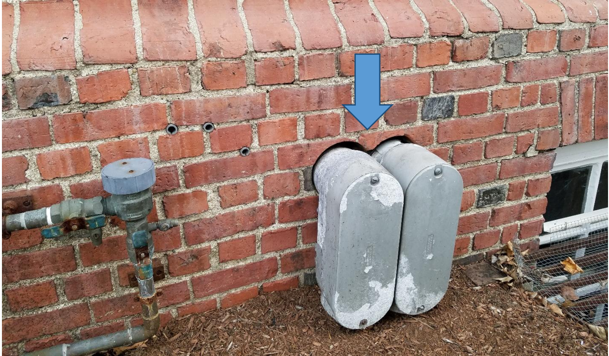
PROVIDE SEALANTS AROUND ELECTRICAL SERVICE PENETRATIONS (WEST)
