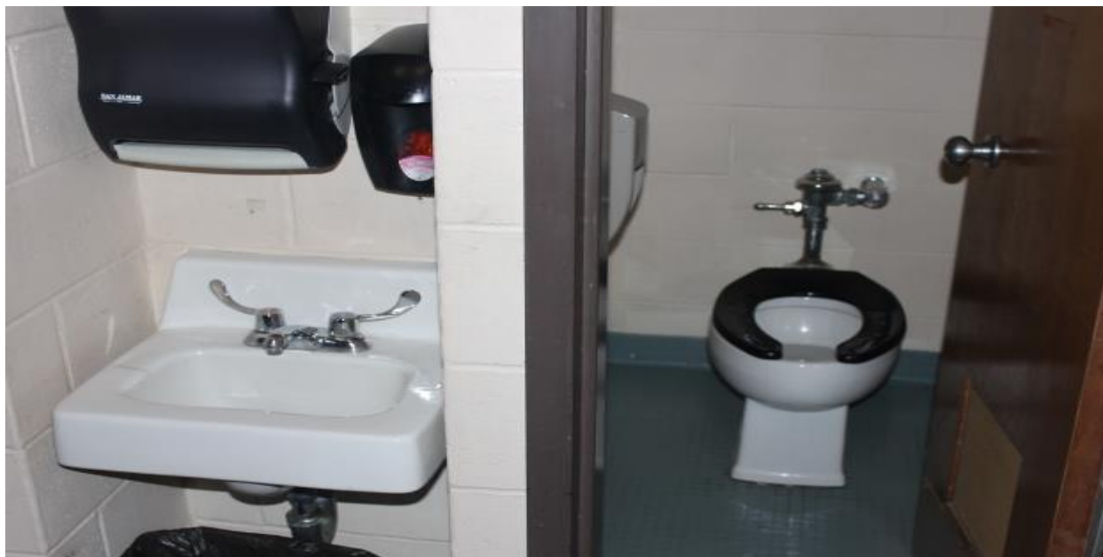
Current undersized bathrooms at classrooms. Non ADA compliant and operationally extremely small.
