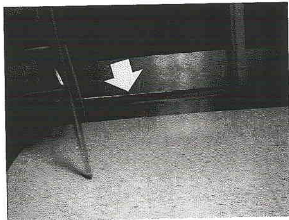
Door Weather Stripping – clear daylight around the door shows a direct pathway for unwanted air leakage.
