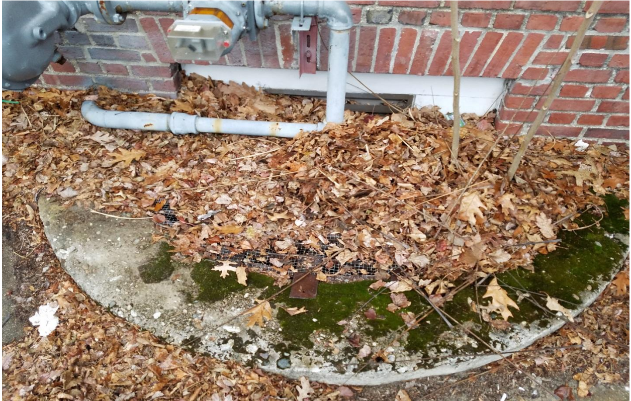
SHOWING AREA WELL DEBRIS BLOCKING MECHANICAL LOUVERS ( REAR )
