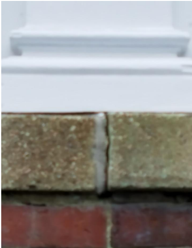
OPEN SILL JOINT TO BE REPOINTED and SEALANT ADDED TO WINDOW SILL ABOVE
