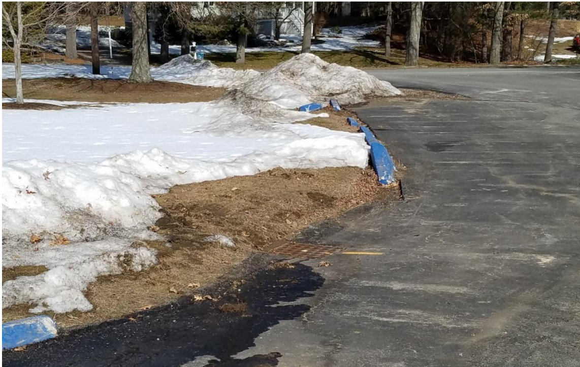
Showing front driveway / parking area with dislodged curb stops and lack of pavement markings
