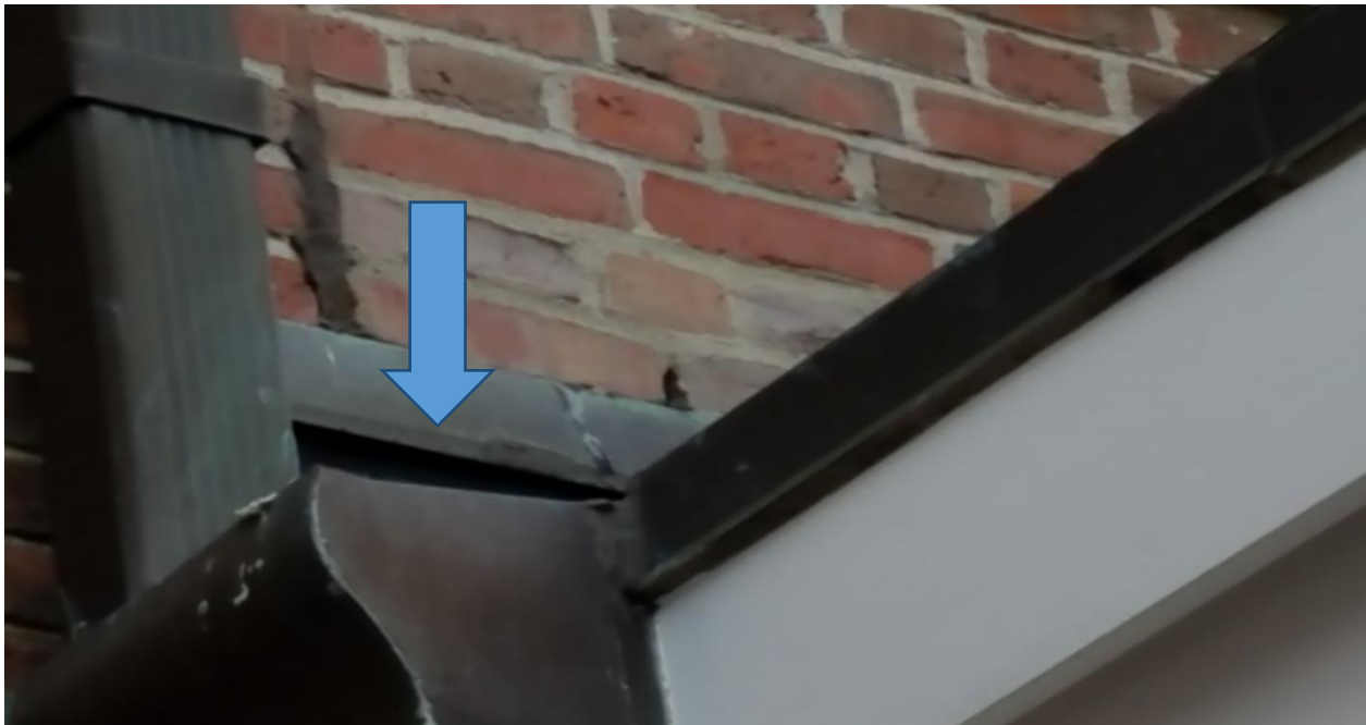
UPLIFTED COUNTER FLASHING (ARROW) ON REAR ELEVATION
