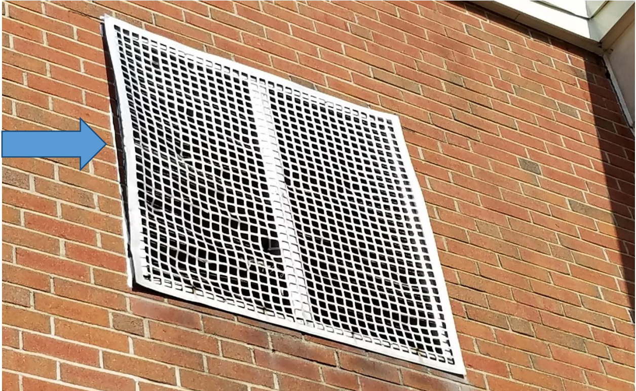
Mechanical louver needing replacement
