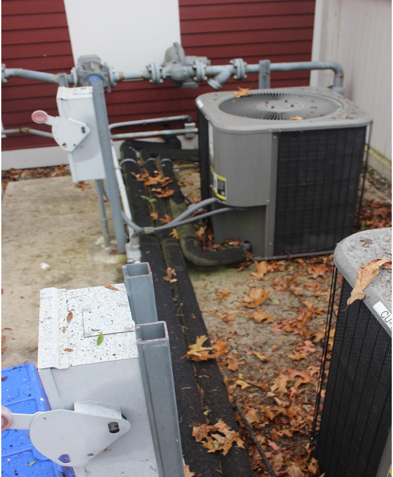
Ground mounted condensing units
