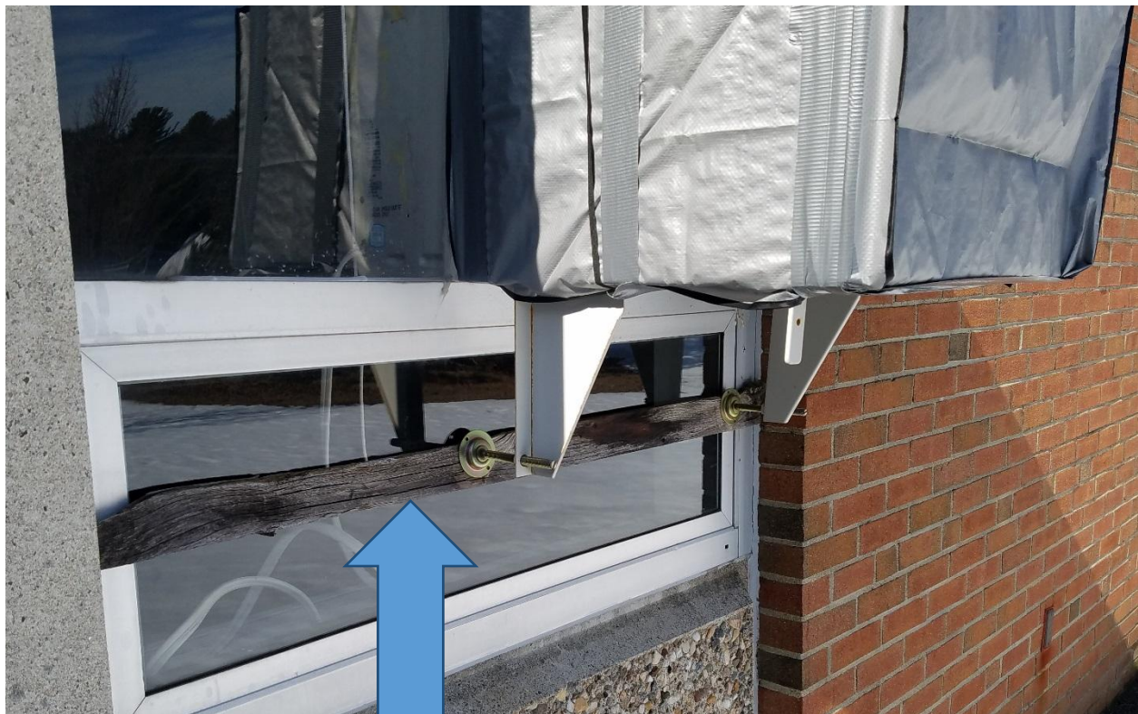
Poor installation of air-conditioner using scrap wood- potential to damage window glass
