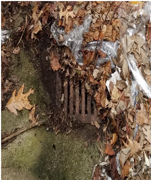
CLOGGED DRAIN IN EXTERIOR STAIRWELL
