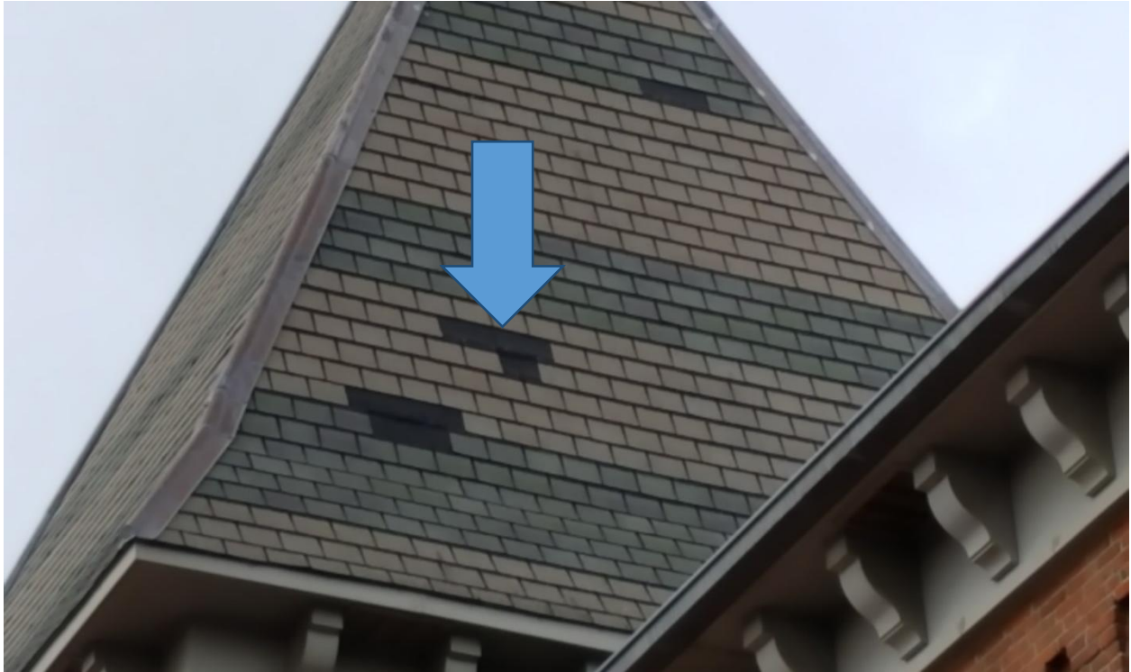
MISSING SHINGLES ON TOWER ELEMENTS
