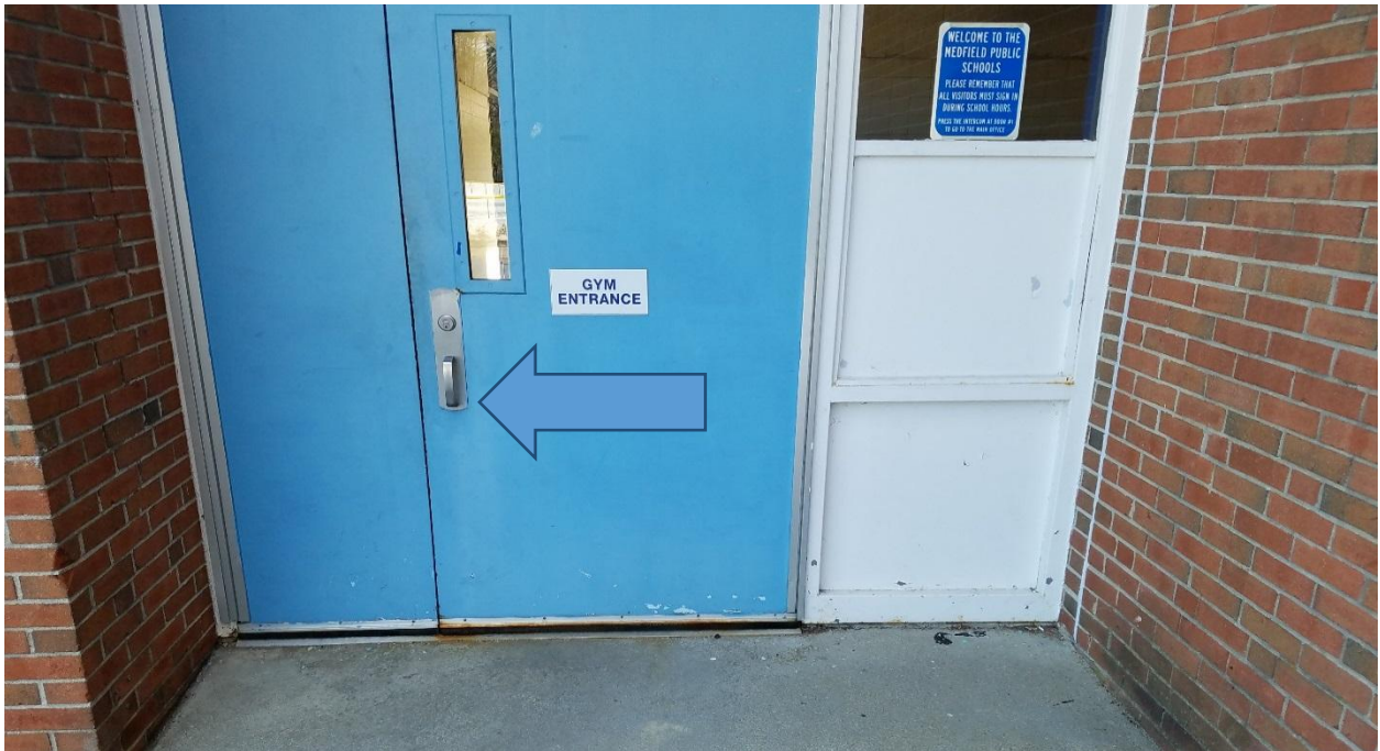
Another example of accessible entrance needing compliant latching hardware
