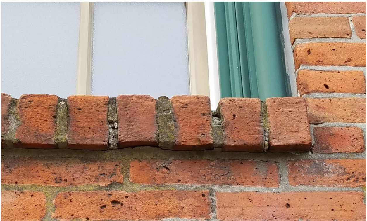
TYPICAL EXAMAPLE OF DETERIORATED ROXLOC BRICK SILLS
