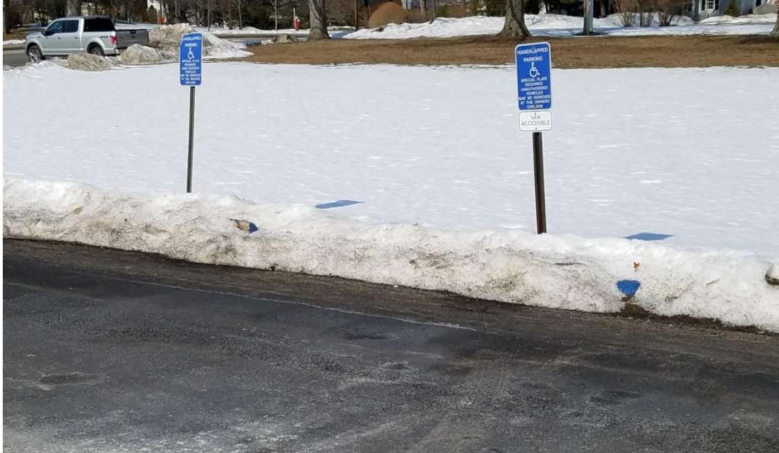
Accessible parking spaces lacking pavement markings & non-compliant sign height
