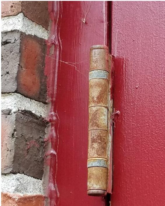
RUSTED DOOR HINGES (SOUTH ELEVATION)
