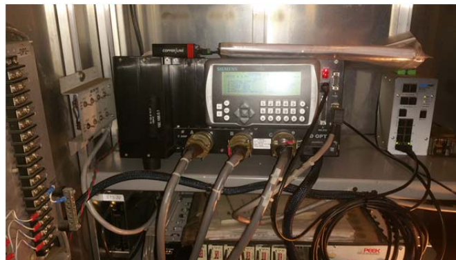
Photo 14. Siemens m50 Traffic Control System at Main Street (Route 109)/Spring Street (Route 27)/N. Meadows Road (Route 27)
