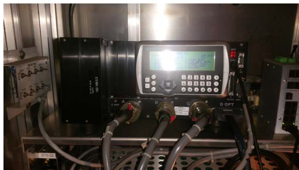
Photo 20. Siemens m50 Traffic Control System at Main Street (Route 109)/South Street
