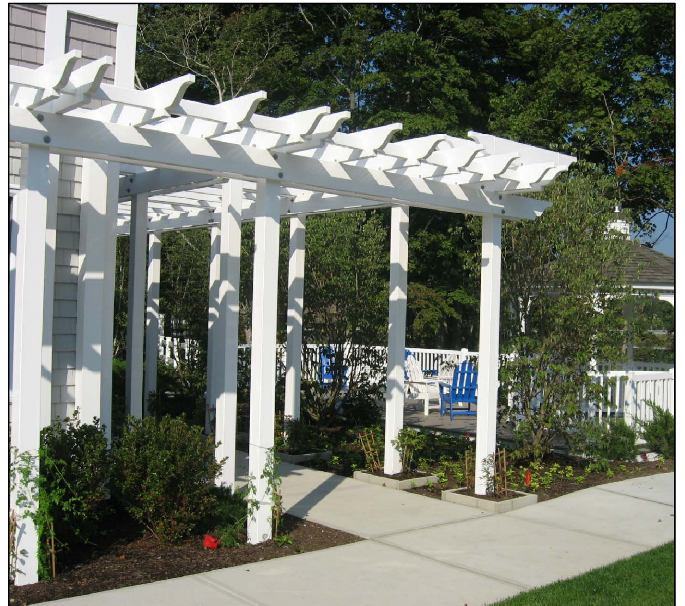
VINYL TRELLIS ASSEMBLIES AT SIMILAR APARTMENT BUILDINGS
