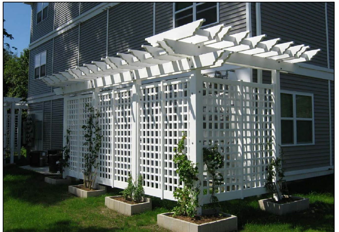
VINYL TRELLIS ASSEMBLIES AT SIMILAR APARTMENT BUILDINGS
