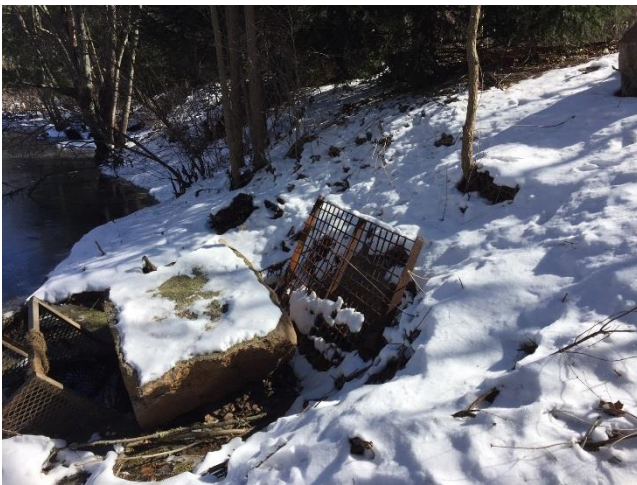
Photo 2: View of western end of box culvert with apparent beaver device.
