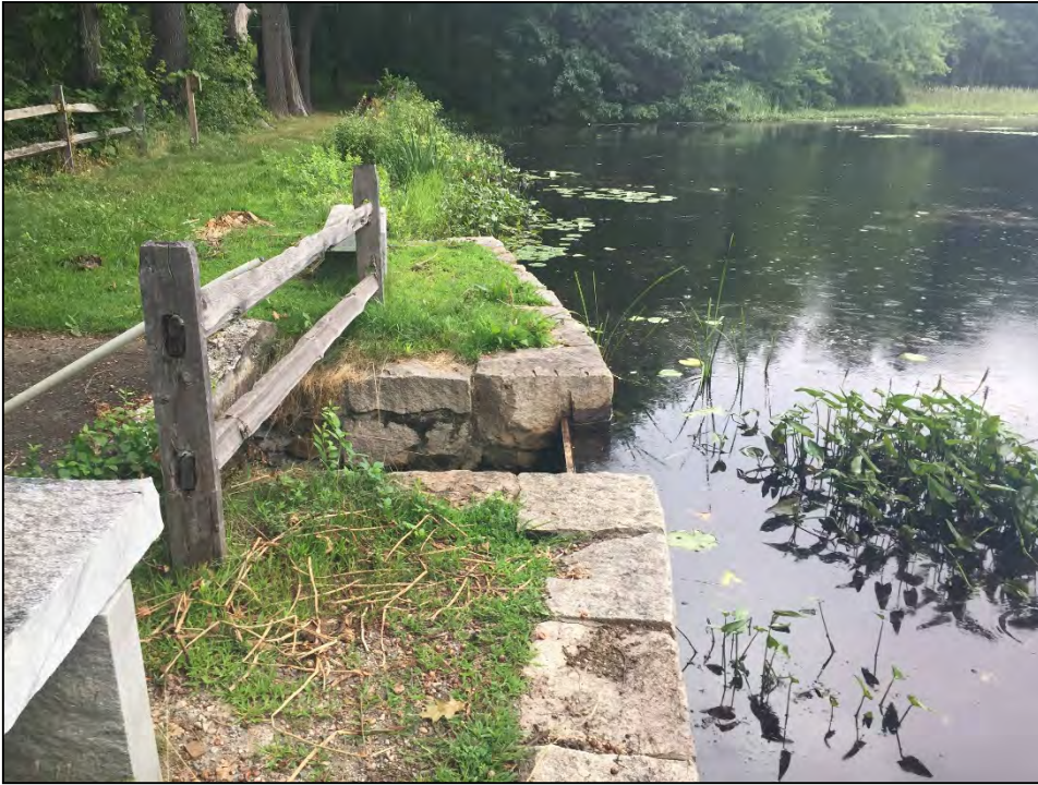
Photo No. 13: Approach and upstream wing/return walls of the spillway.
