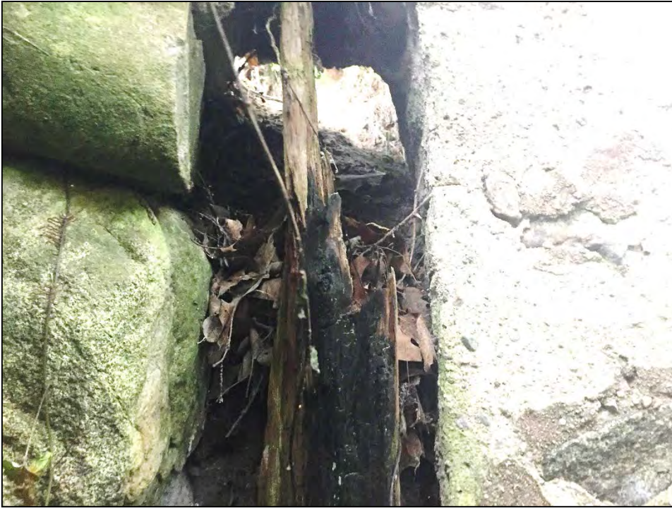
Photo No. 21: View of the erosion of the ground surface behind the left training wall at the transition between the stone masonry and concrete sections. Note deteriorated timber at transition.
