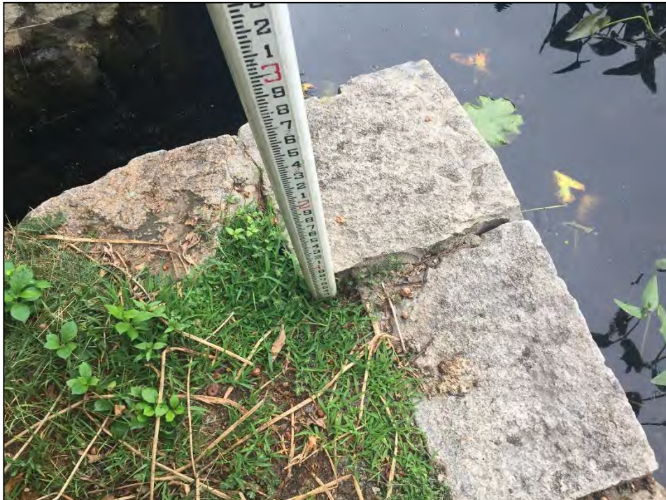
Photo No. 16: 6-inch diameter by 6-inch deep potential subsidence behind the upstream end of the left training wall.
