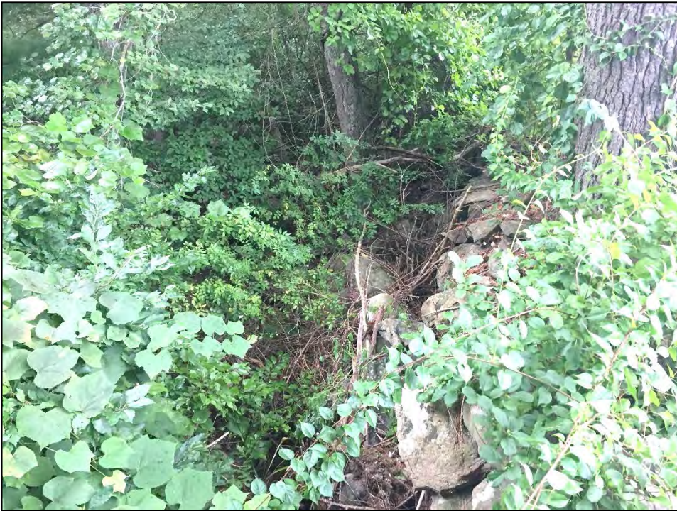
Photo No. 11: Failed/failing sections of the irregular stone masonry wall along the downstream side of the dam right of the spillway. Typical several locations. Note soft and saturated ground surface with wetland vegetation within the downstream area.
