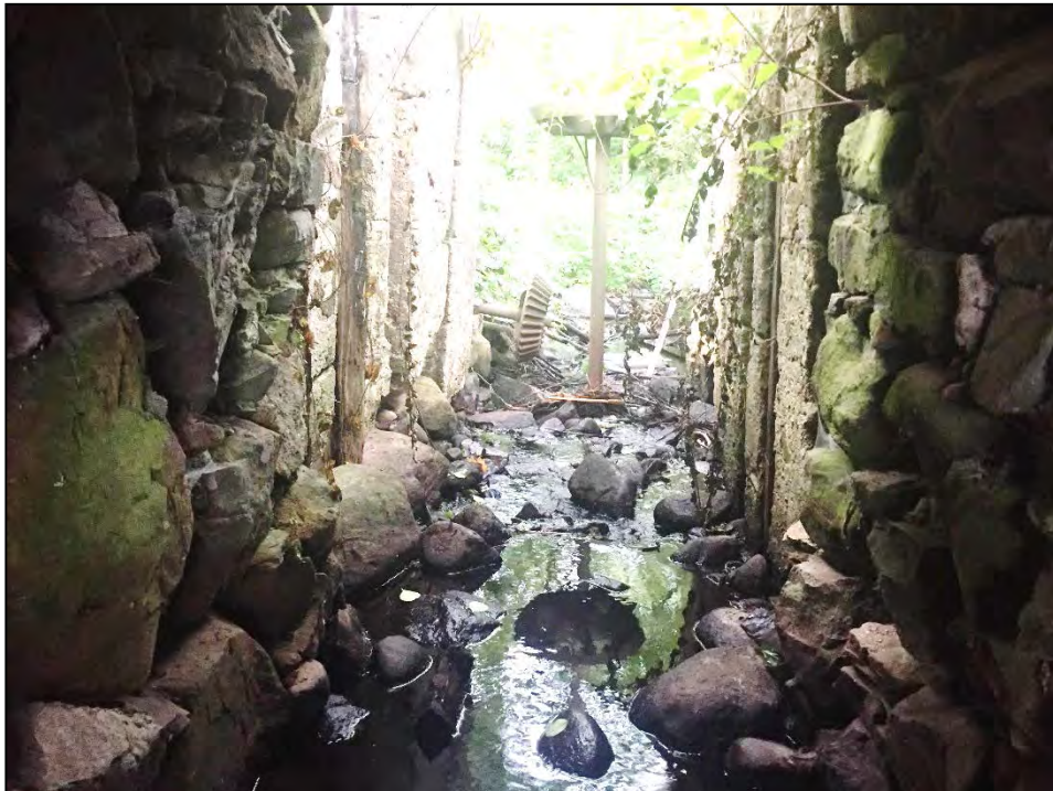
Photo No. 18: Spillway channel from 5 feet downstream of the spillway looking downstream. Note transition to concrete walls at approximately 20 feet downstream of the spillway controls.
