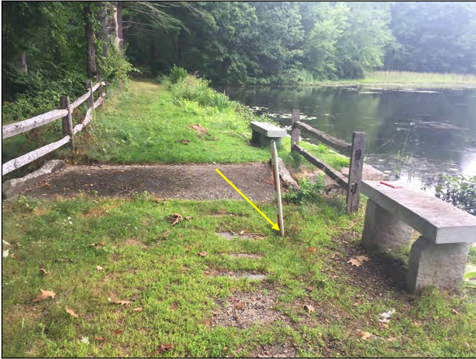
Photo No. 17: 12-inch diameter by 12-inch plus deep subsidence/sinkhole located 5 feet downstream and 3 feet left of the left training wall (Yellow Arrow).
