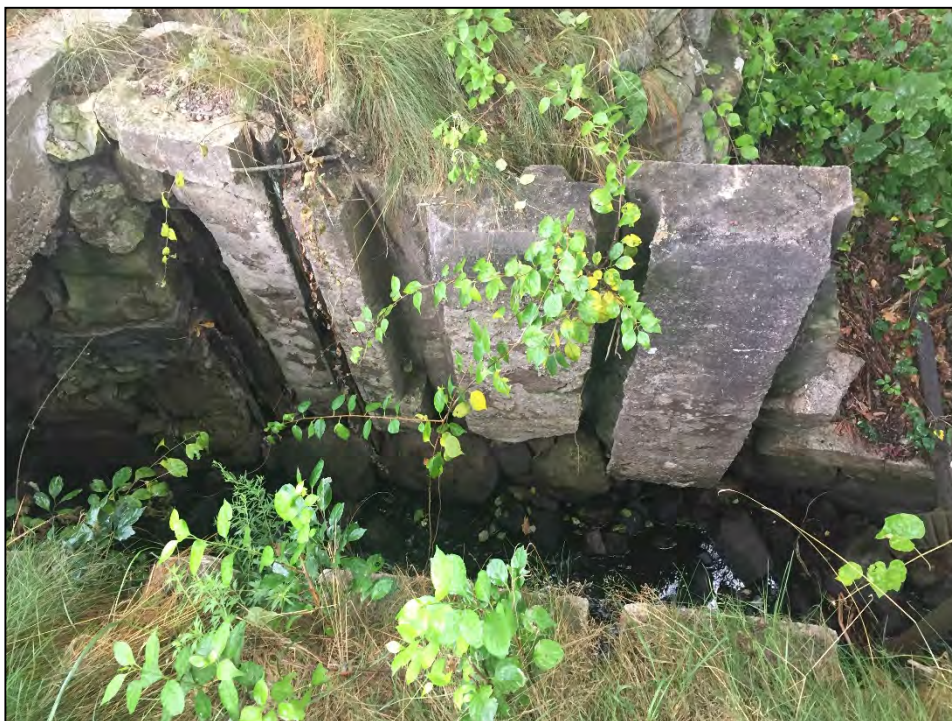
Photo No. 20: Left concrete training wall. Note significant deterioration and apparent displacement of the wall. Right wall is similar
