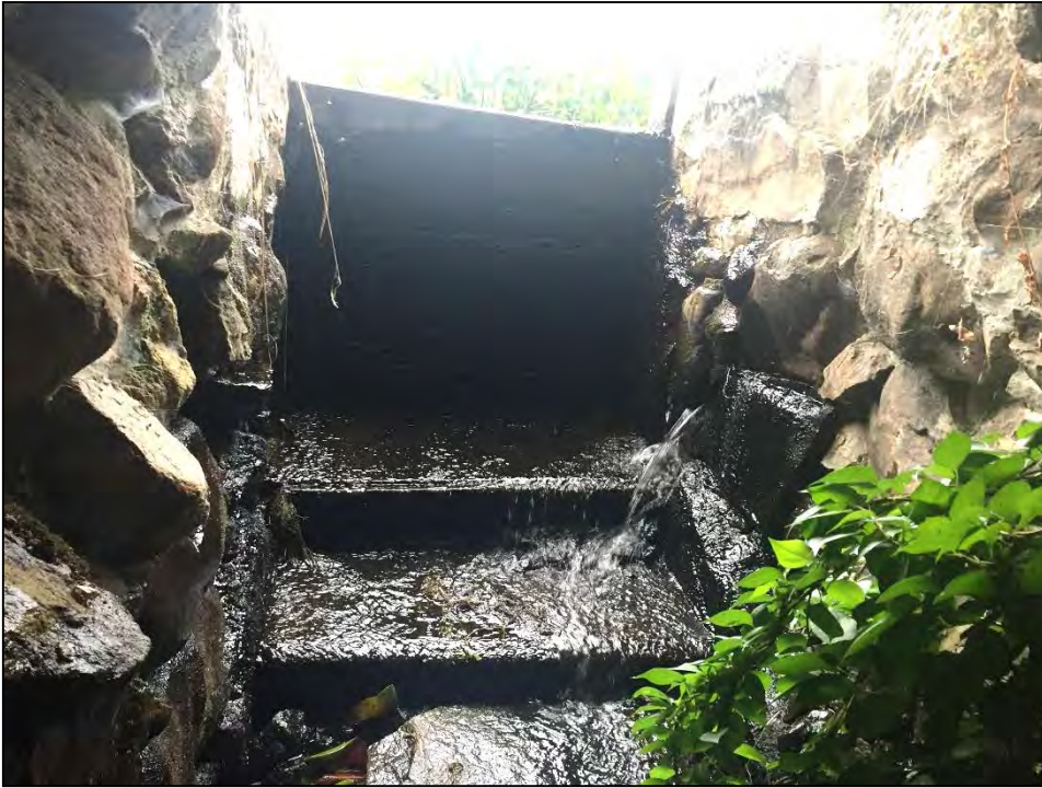
Photo No. 15: Leakage from the left and right training walls of spillway channel. Note the highest area of leakage from the left wall approximated at 20-30 GPM.
