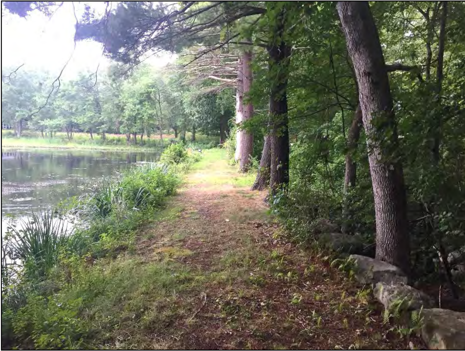
Photo No. 7: Crest near the right abutment looking left. Note large diameter trees along the top of the downstream side of the dam.
