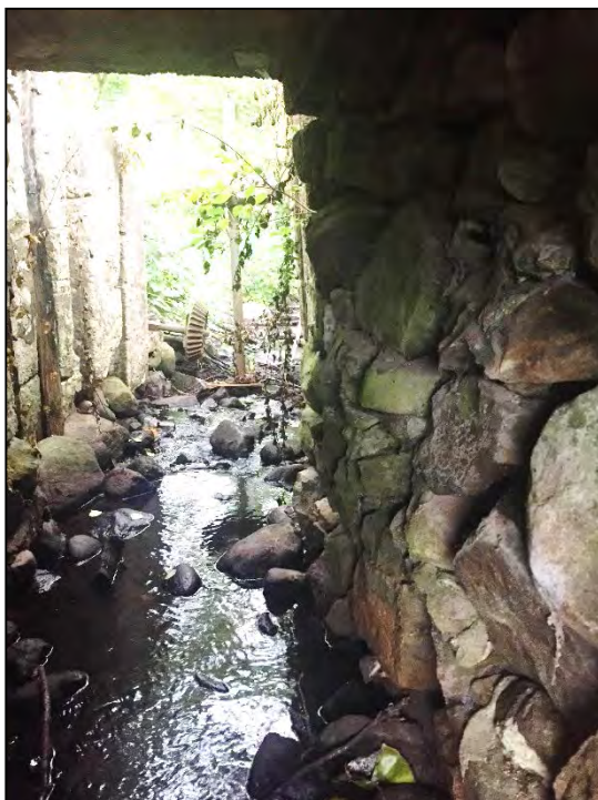
Photo No. 19: Potential bulge in the downstream portion of the right training wall within 5 feet of the transition to the concrete wall.
