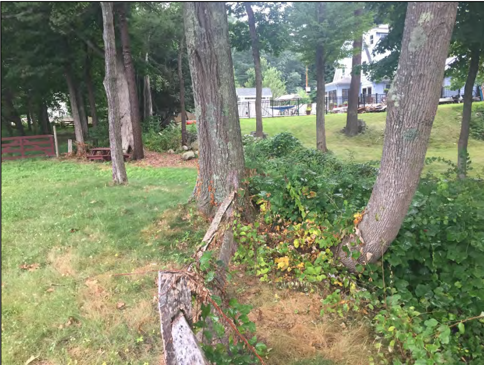
Photo No. 8: Downstream side of the dam from the spillway looking left. Note large diameter trees and underbrush limiting the inspection in this area.
