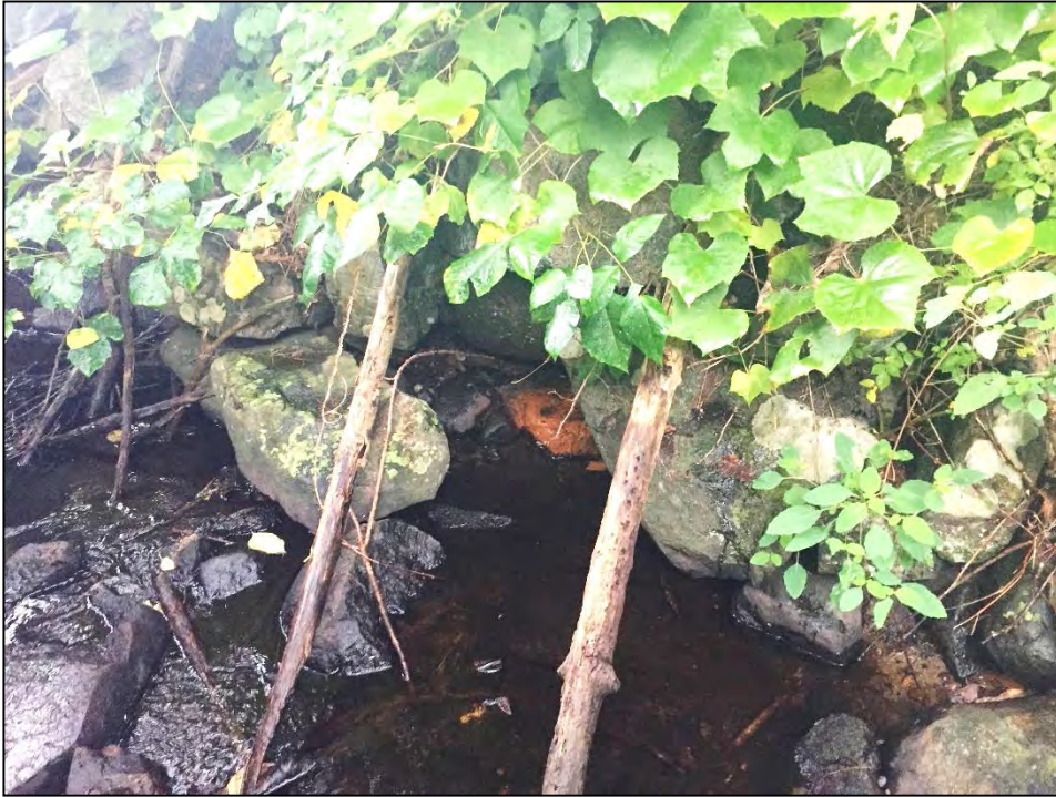
Photo No. 9: Iron oxide staining at toe of the downstream wall immediately left of the spillway downstream channel.
