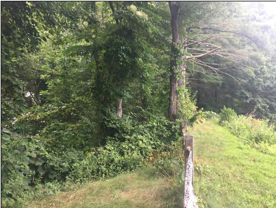
Photo No. 10: Downstream side of the dam from the spillway looking right. Note large diameter trees and thick underbrush that limited the inspection of this area.
