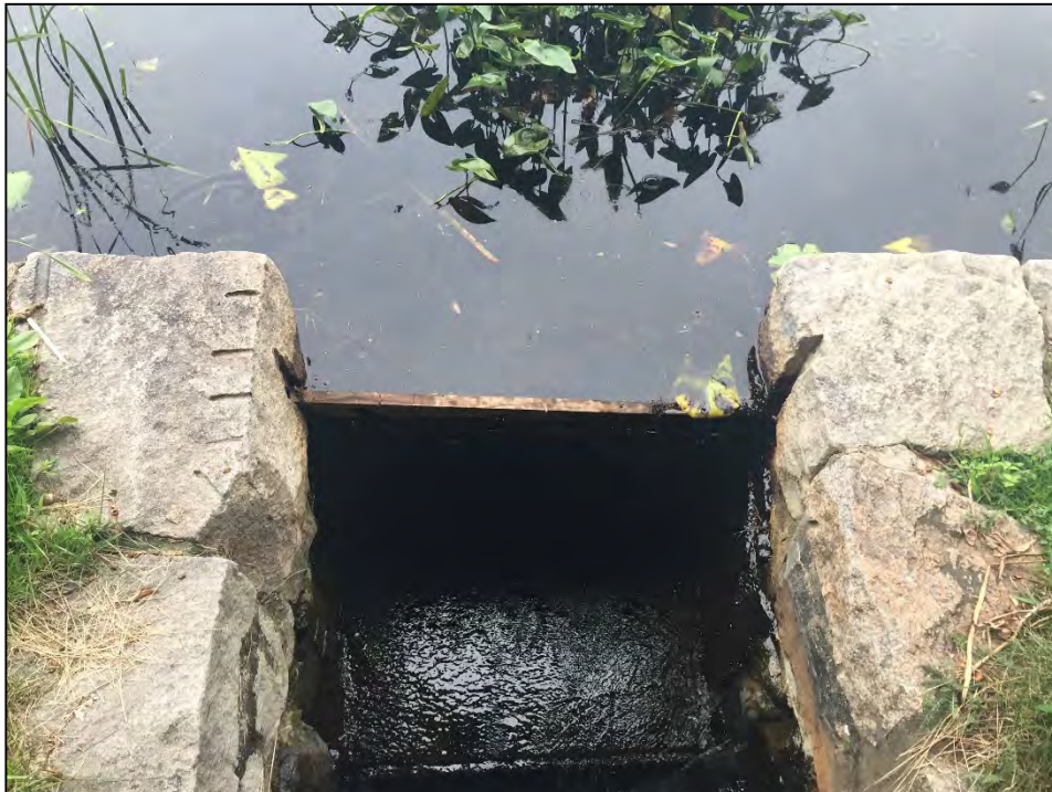
Photo No. 14: Spillway stops logs and stepped concrete invert.
