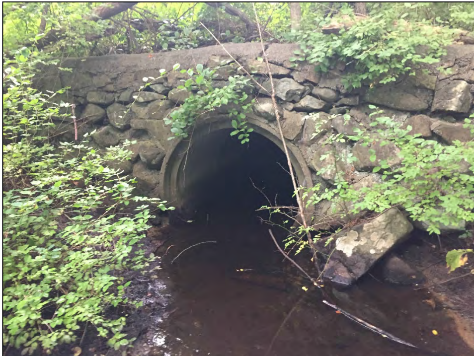
Photo No. 24: View of the 4-foot diameter RCP culvert that extends under Homestead Drive.
