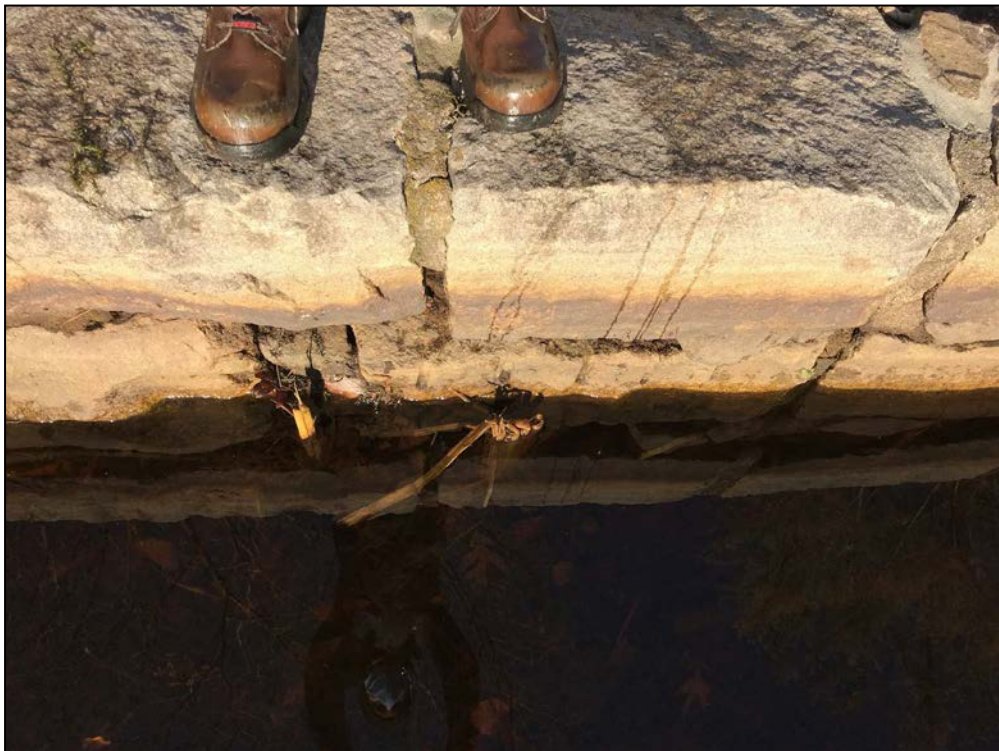
Photo No. 8: Typical upstream wall joint condition right of the spillway.
