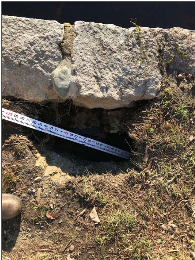
Photo No. 10: Sinkhole behind upstream right wall probed to 2.6 feet left of the sinkhole.
