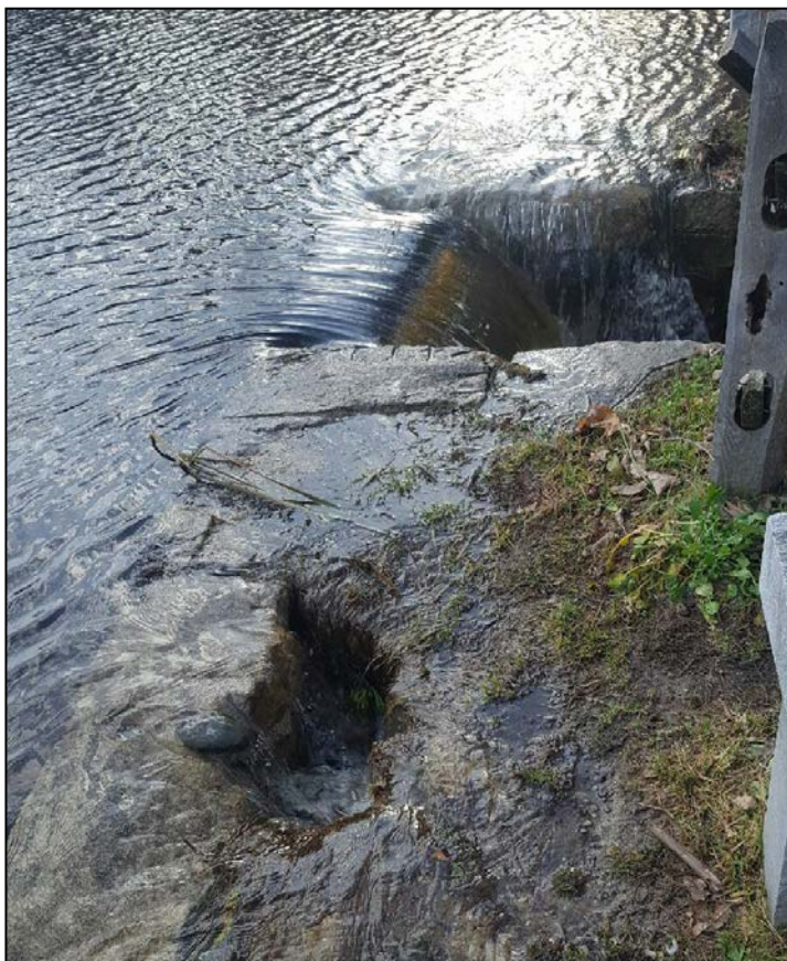
Photo No. 14: Flow overtopping training walls (Taken on 12/1; provided by Town).
