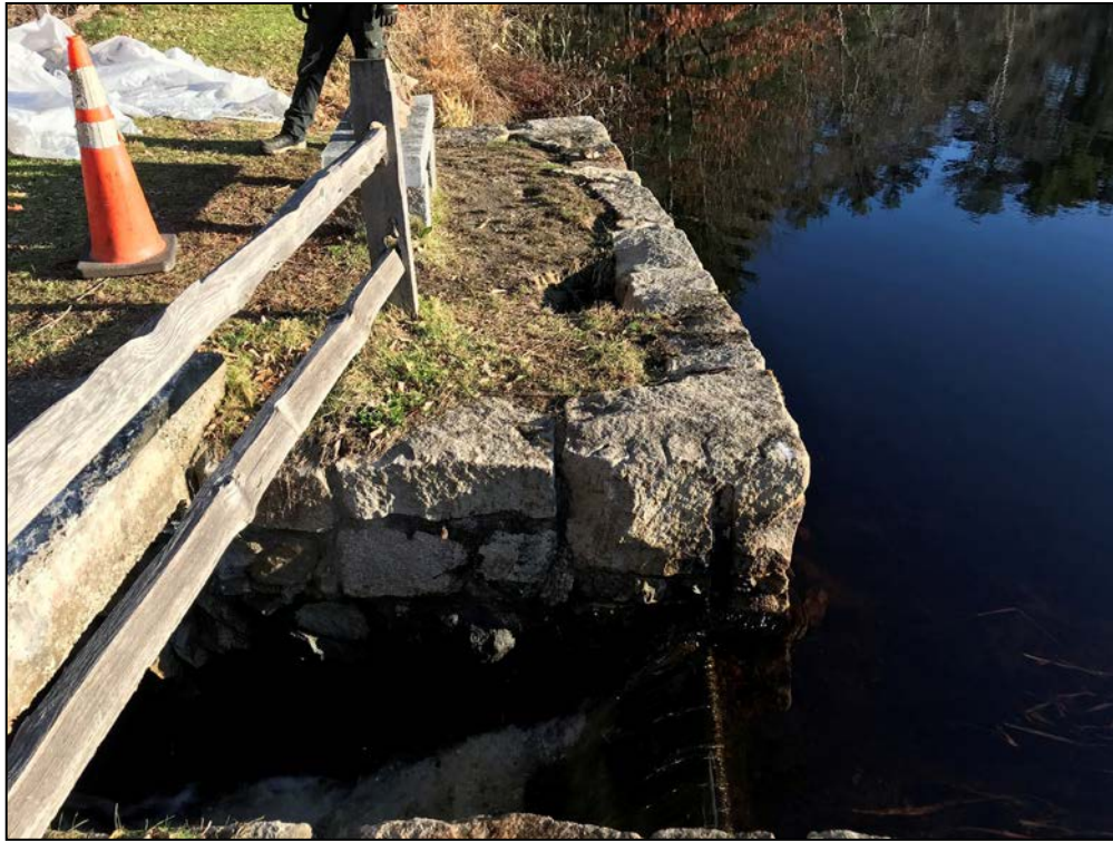
Photo No. 7: Right side of the spillway. Note sinkhole behind upstream wall.
