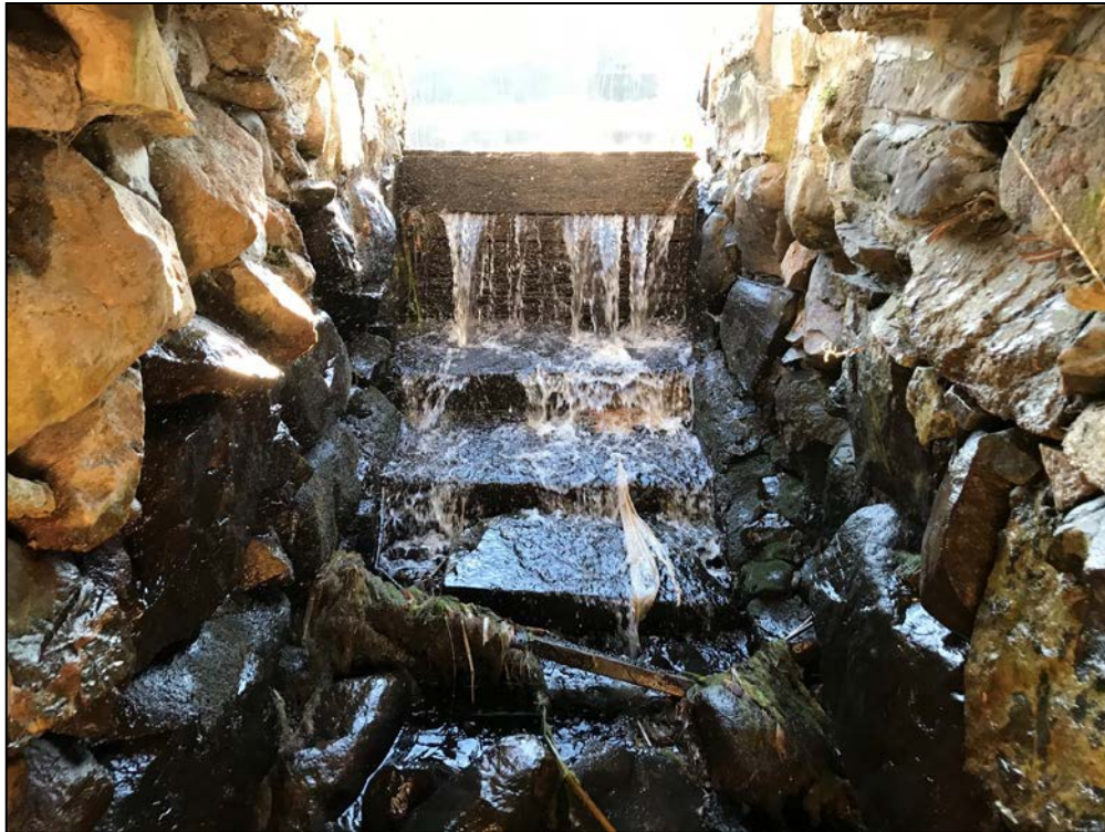
Photo No. 11: Downstream side of spillway (Note: Stoplog installed to stop flow and allow for inspection).
