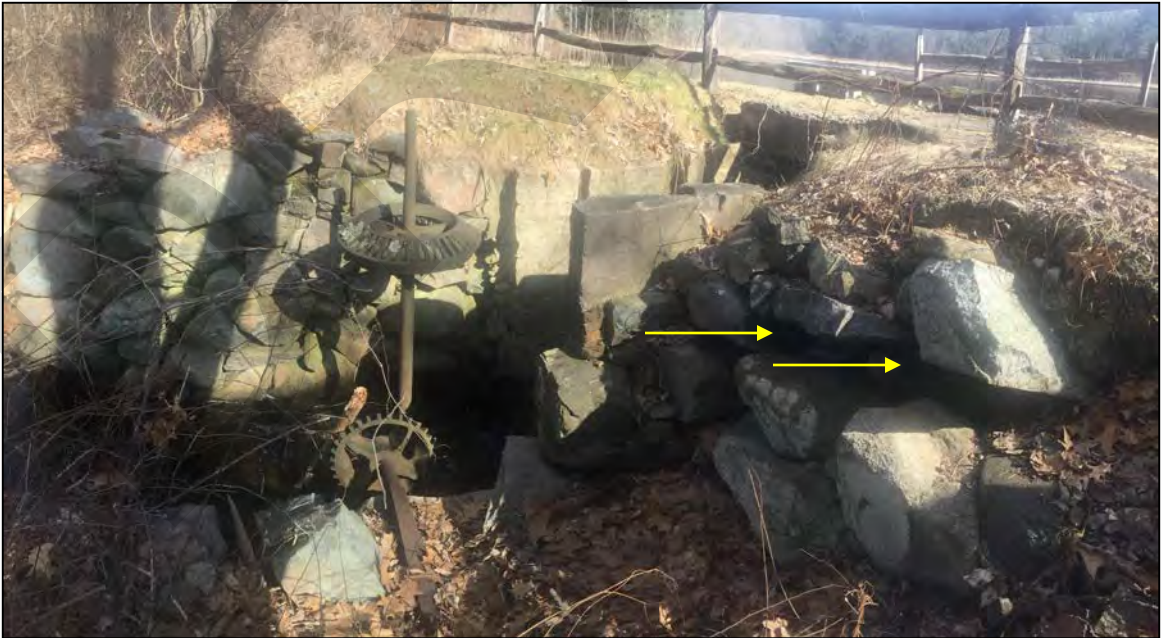
Photo No. 14: Overview of the primary spillway discharge and downstream walls. The left wall has at least two voids up to 42 inches deep.
