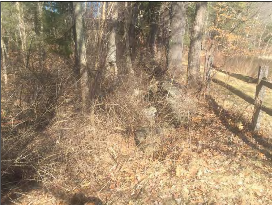
Photo No. 6: Downstream slope as viewed from near the primary spillway looking right. Note the overgrowth of trees, brush, vines, and briars.
