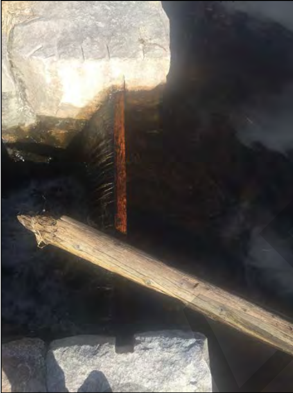
Photo No. 11: Primary spillway stop log section.
