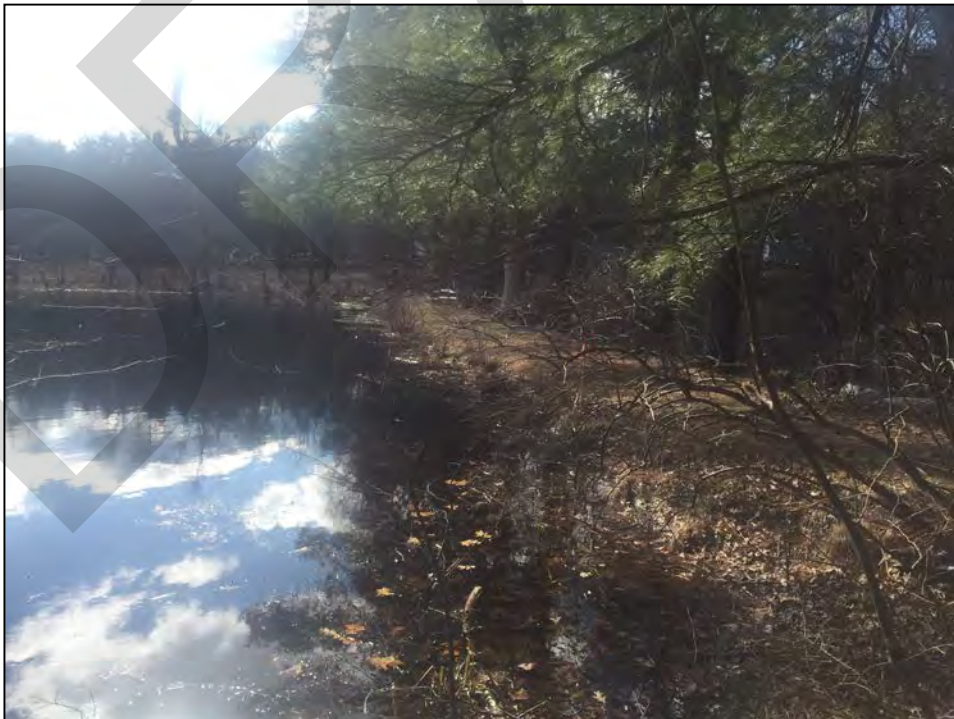
Photo No. 4: Overview of the upstream side of the dam as viewed from the right abutment looking left. Note the irregular shoreline due to scarping, and brush growth.
