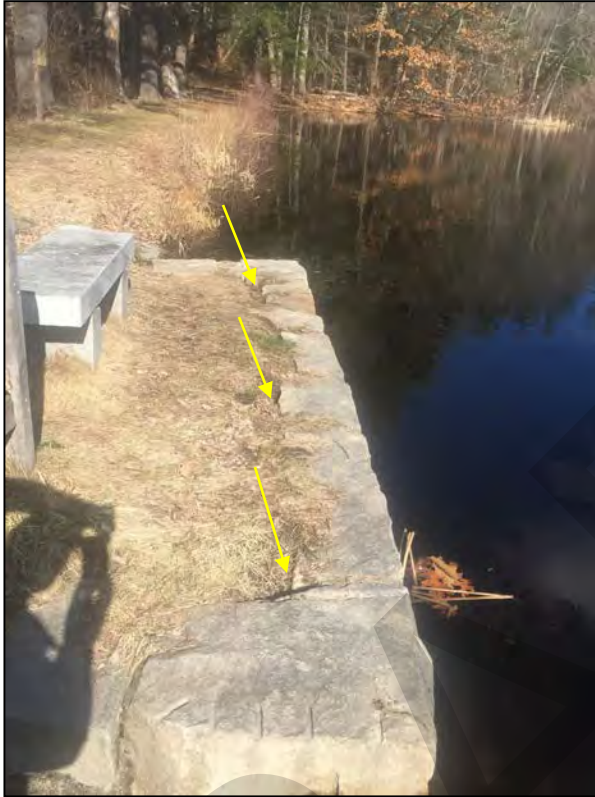
Photo No. 3: The upstream side of the dam as viewed from the primary spillway looking right. Note the sinkholes forming behind the spillway right return wall and the irregular shoreline beyond.
