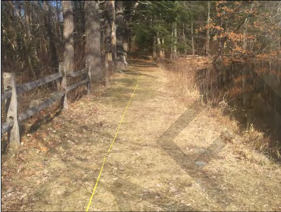
Photo No. 5: Crest as viewed from near the primary spillway looking right. Note the large trees along the downstream edge.
