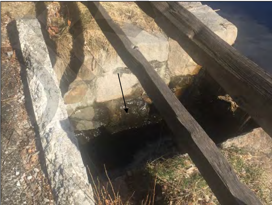
Photo No. 12: Primary spillway right training wall downstream of stop logs. Note seepage/leakage.
