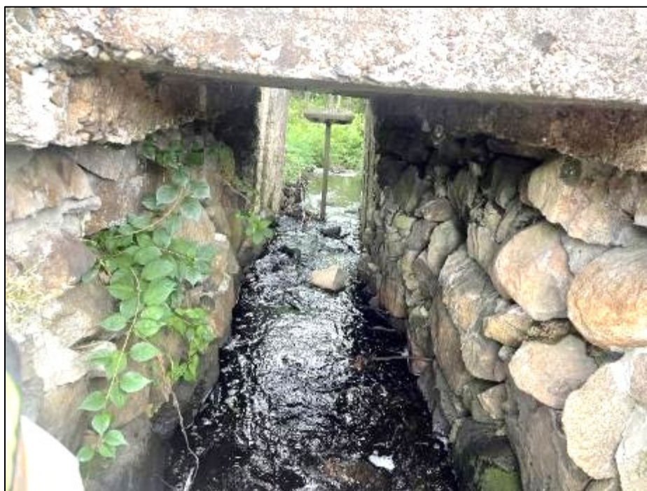
Photo No. 12.: Discharge channel of the spillway from the control section looking downstream.
