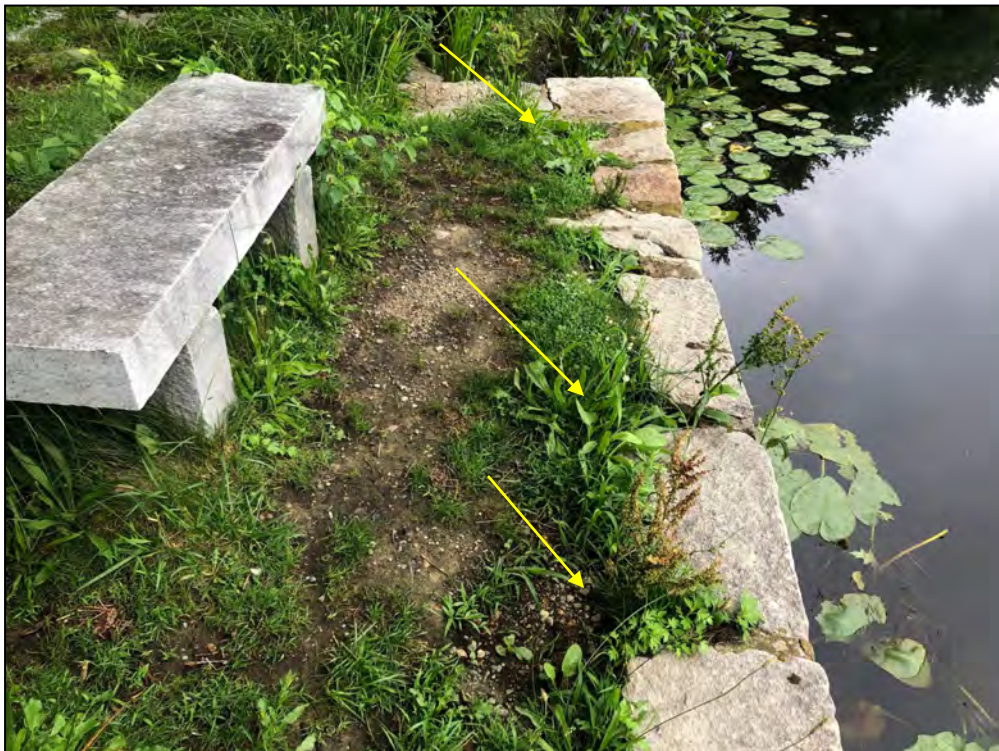
Photo No. 6: Upstream wall from the spillway looking right. Note arrows pointing to sinkholes behind wall.
