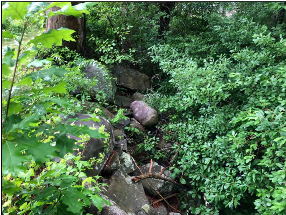
Photo No. 16: Downstream slope from near STA 1+75 looking left. Note irregular wall that appears to be failed.
