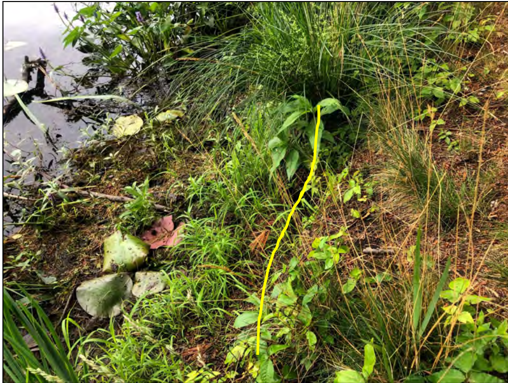
Photo No. 7: Scarping on the unprotected section of the upstream slope, near STA 2+00.
