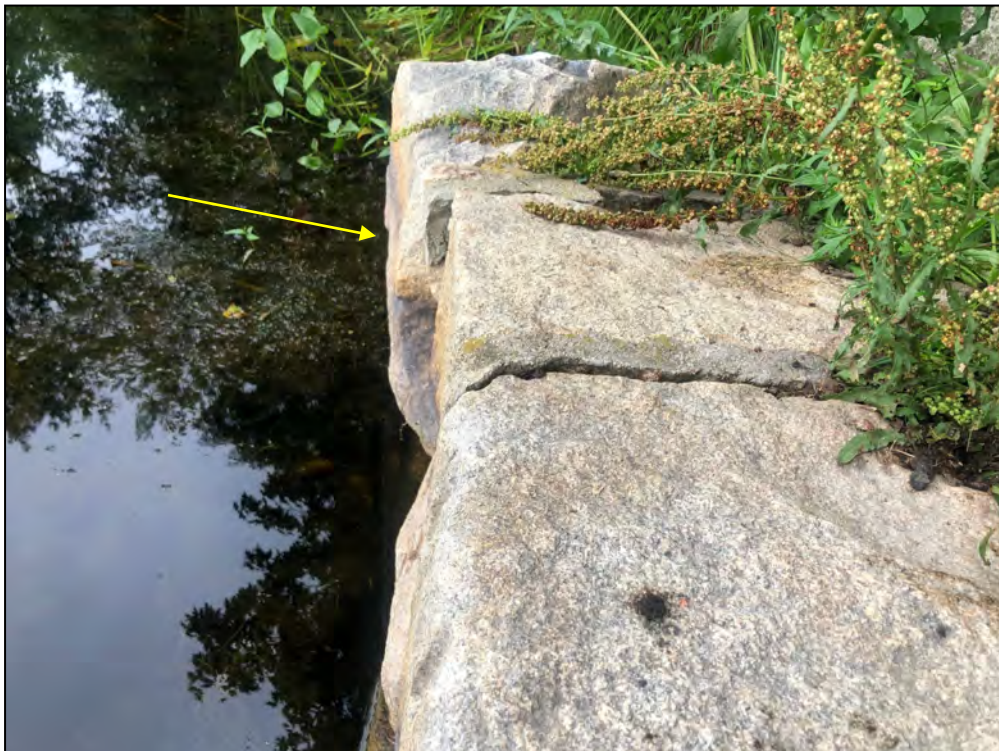
Photo No. 4: Left end of the upstream wall. Note movement of the wall towards the impoundment.
