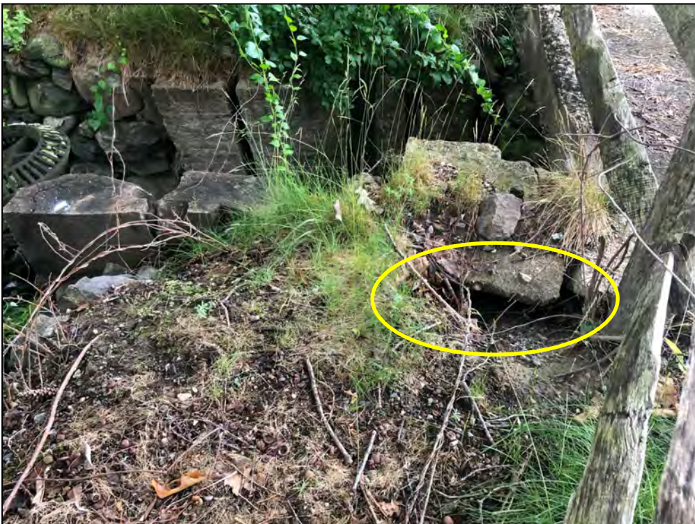
Photo No. 22: Surface behind the left downstream training wall. Note apparent subsidence and sinkhole.
