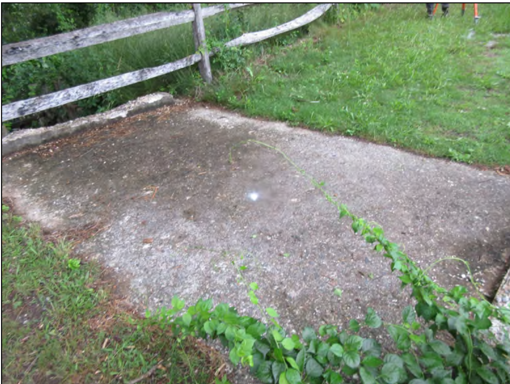
Photo No. 10: Concrete slab over the spillway near STA 0+85.
