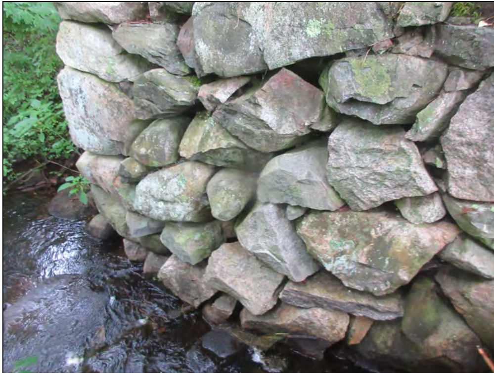
Photo No. 23: Right downstream stone training wall. Note voids between the stones.
