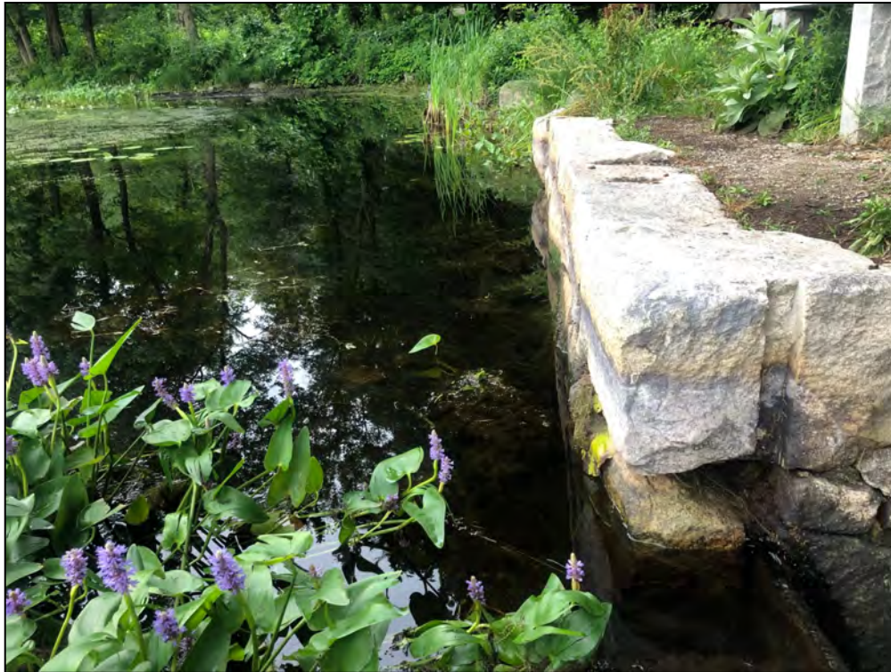
Photo No. 5: Upstream wall from the spillway looking left. Note voids within the wall.
