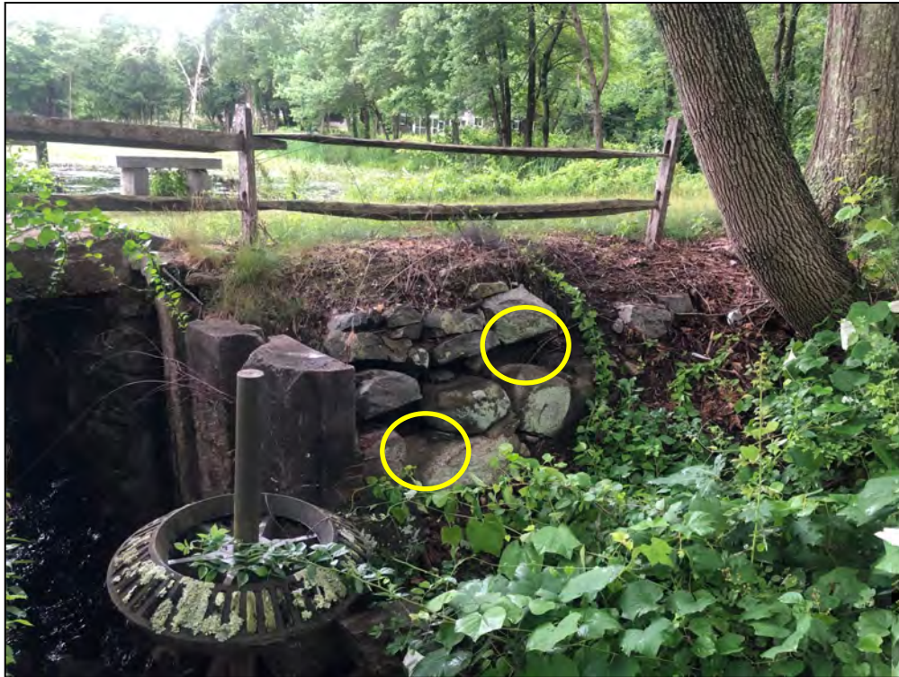
Photo No. 15: Stone wall to the left of the spillway. Note large voids that were probed to 48-inches.
