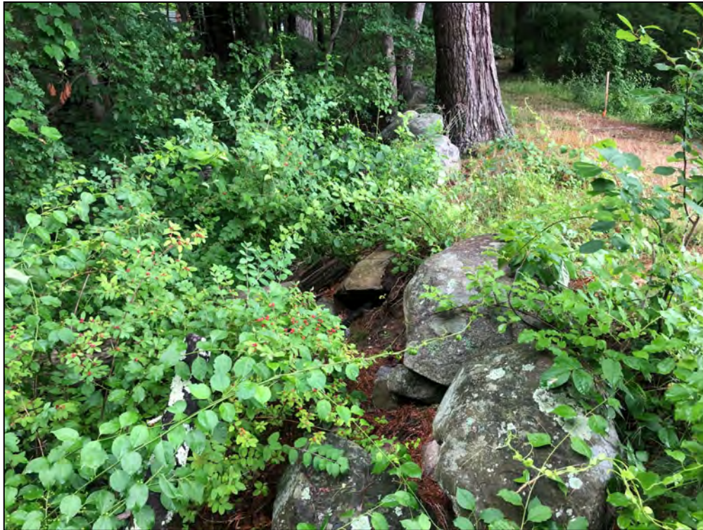
Photo No. 17: Downstream slope from near STA 1+75 looking right. Note large tree at top of slope.
