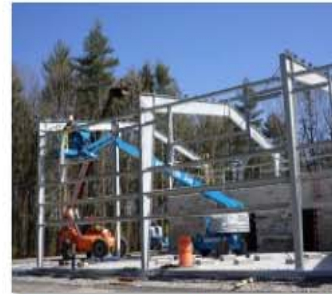
Wall framing and diagonal bracing at A-line.JPG
