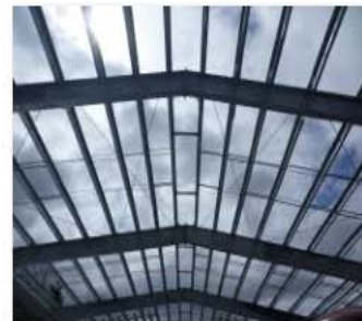
Diagonal roof bracing in place.JPG
