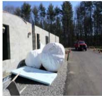
Chemical bulk tanks.JPG
