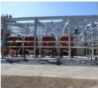
Filter tanks set in place.JPG
