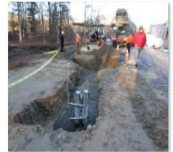
Concrete placement at duct banks.JPG
