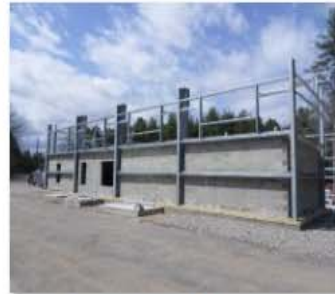
Structural Steel at D line..JPG
