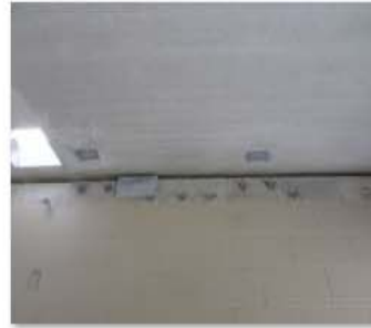
Seismic clips at precast planks.JPG
