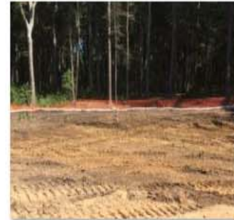
Erosion Controls - WTP.JPG
