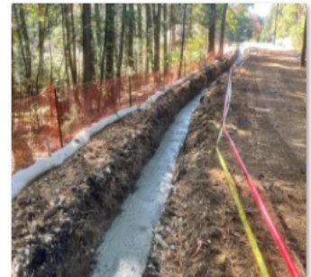
10.18.21 Access Road Elec Trench.jpg
