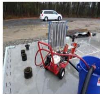
Pressure testing 4 PVC force main.JPG
