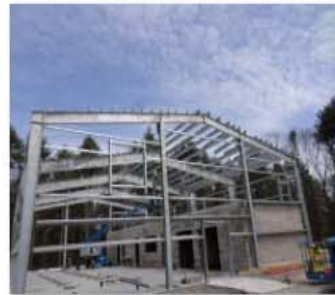
Wall framing amd roof purlins at West wall.JPG
