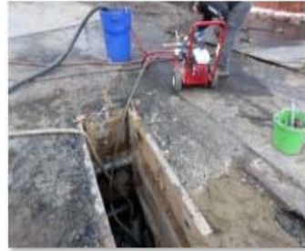
11.29.2021 WM Pressure Testing.JPG
