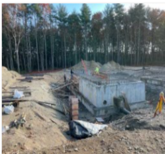
11.15.2021 Backwash Waste Tank Walls (2).jpg
