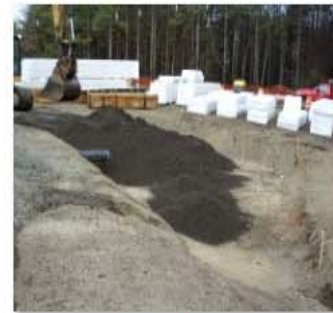
Placing engineered soil at Biobasin #1 (1).JPG
