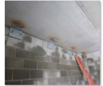
Seismic clips welded to precast planks.JPG
