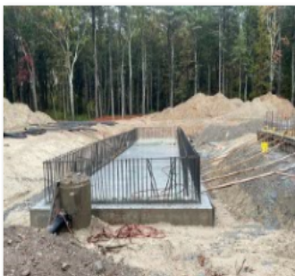
10.25.21 Backwash Waste Tank Slab.jpg
