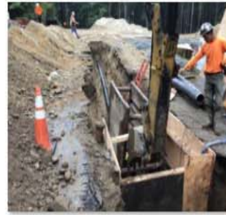
Raw Water Main Installation.jpg
