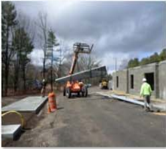
Shaking out structural steel.JPG
