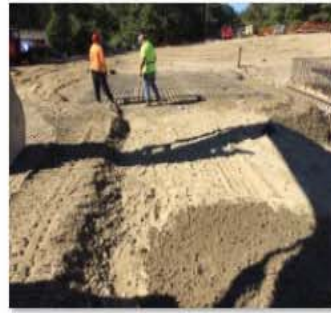
WTP Building Formwork.jpg
