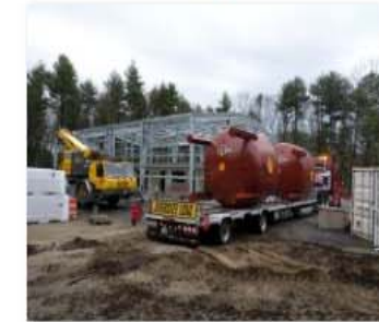
Filter tanks delivered to the site..JPG
