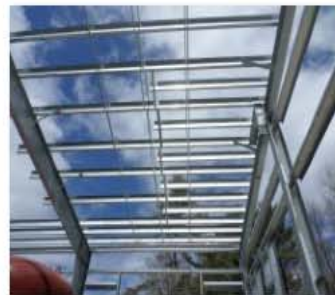
Wind uplift purlins and bridging at 4 to 5 lines.JPG
