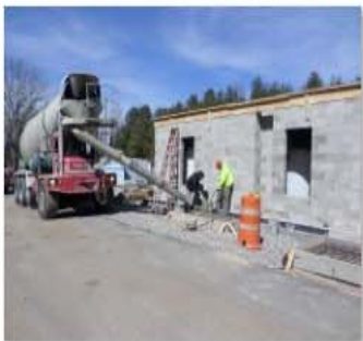
Concrete placement at equipment pads.JPG
