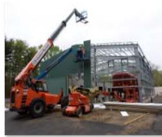
Siding installation at the East elevation.JPG
