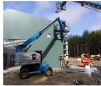
Siding panels at the North East corner.JPG
