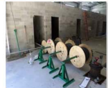
Installation of feeder cables.JPG
