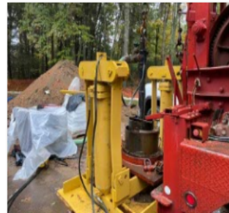
Well 3A Installation.jpg
