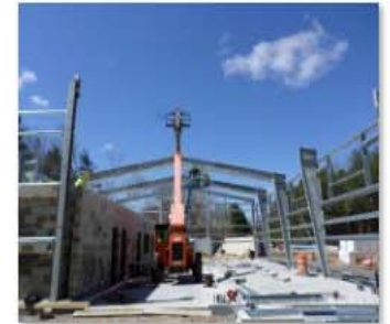
Setting roof rafter at 3 line.JPG
