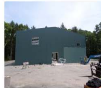
Siding complete West Elevation.JPG
