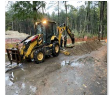
10.25.2021 Elec Trench to Well 3.jpg
