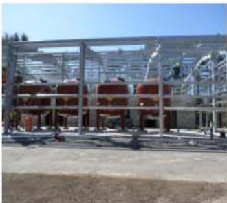
Filter tanks set in place.JPG
