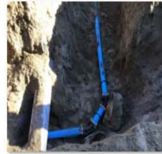
Sewer Forcemain Installation.jpg
