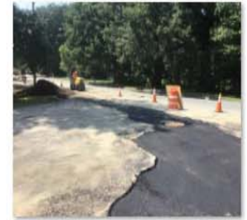
Photo 1 - Elm St Paving.jpg
