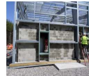
Installation of window trim at the NaOH room..JPG
