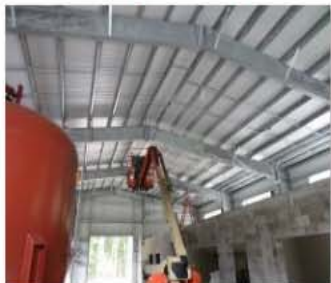
Roof panels complete.JPG
