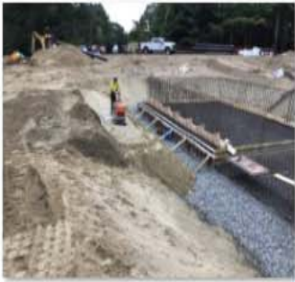
Backwash Waste Tank Formwork.jpg
