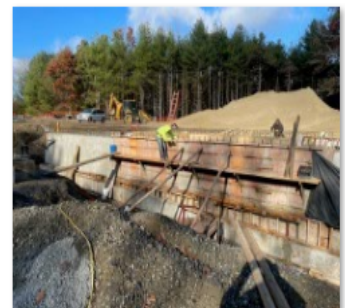
11.15.2021 Backwash Waste Tank Walls.jpg
