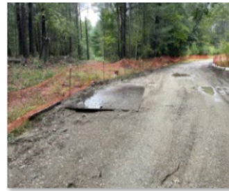
10.4.21 Well 4 Access Road.jpg
