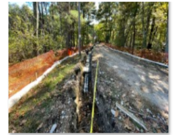
10.18.21 Well 3 Access Road Elec Trench.jpg
