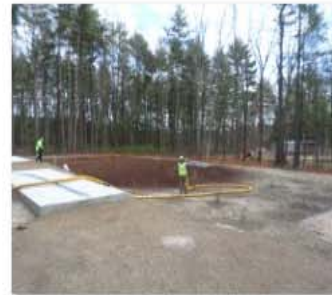
Spreading mulch at Bio Basin 2..JPG
