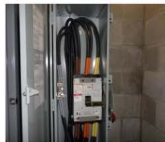
Terminating cables at generator breaker (1).JPG
