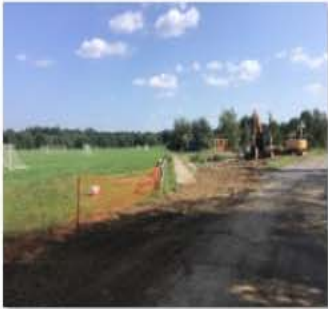
Photo 2 - Access Road Fencing.jpg
