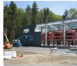
Siding installation at the North elevation.JPG
