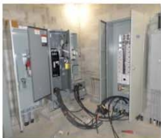
Pulling cable at switch gear.JPG
