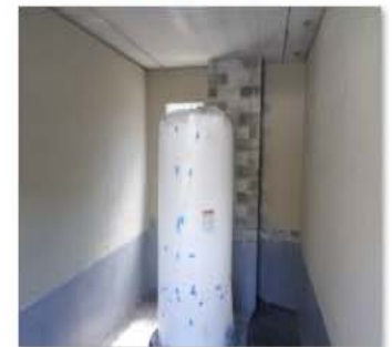
CMU block filler at NaOCL room.JPG
