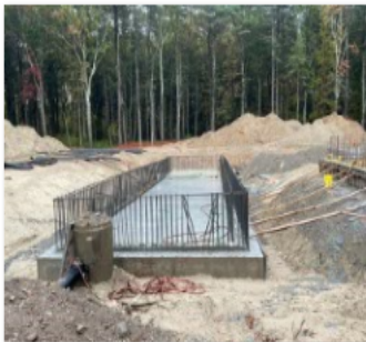
10.25.21 Backwash Waste Tank Slab.jpg
