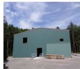
Rake trim installation at West elevation. (1).JPG
