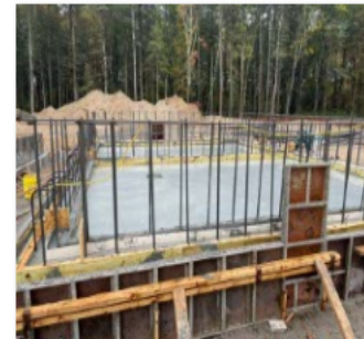
10.25.2021 Chemical Containment Slab.jpg
