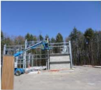
Structural Steel on 1 line..JPG
