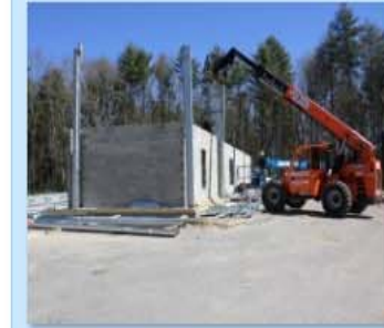
Setting columns at D line..JPG
