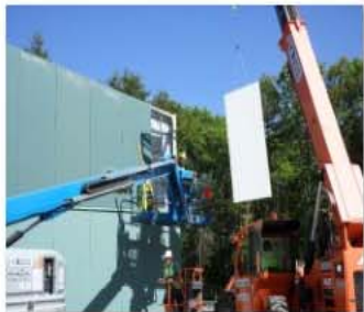
Final wall panel installation.JPG
