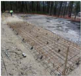
Reinforcing at the propane tank pad.JPG
