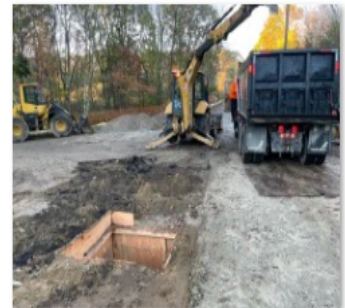
11.01.21 Well 3 Access Road.jpg
