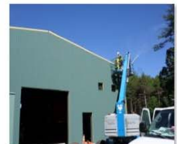
Rake trim installation at East elevation. (2).JPG
