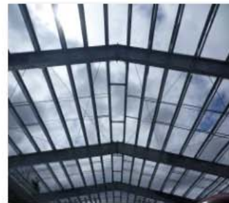
Diagonal roof bracing in place.JPG
