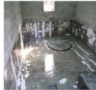
Chemical resistant coating.JPG
