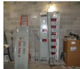
Installation of MCC.JPG
