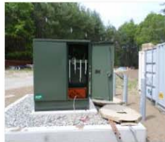
Transformer installation.JPG
