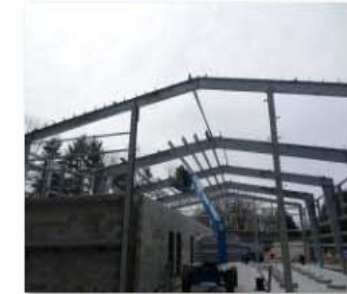
Installation of purlins at the South side of the building..JPG
