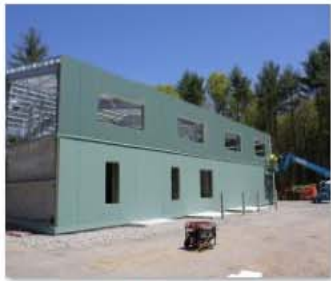
Siding panels at the South side of the building.JPG
