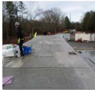
Grouting keyways at precast planks.JPG
