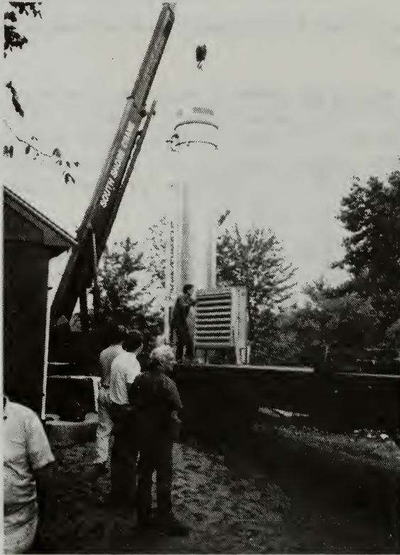
Installation of the aeration tower for wells 1 & 2 on Route 109
