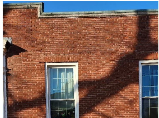
Typ. South Wall Lintel Corrosion & Cracking
