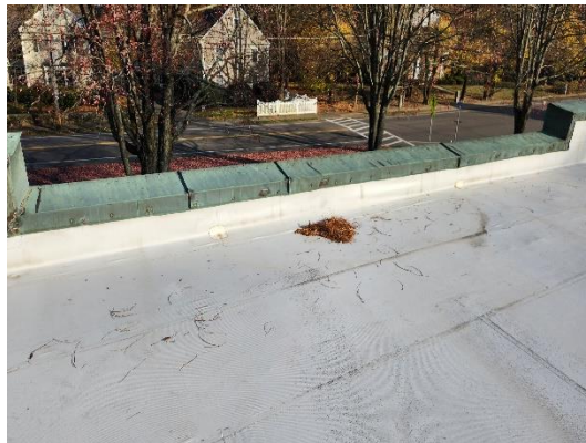
Typical view of EPDM Roofing
