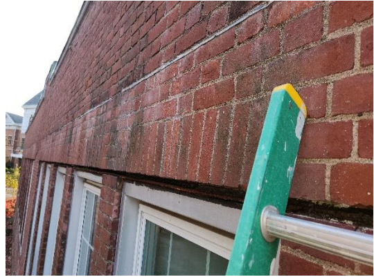
Typical East Wall Lintel Corrosion
