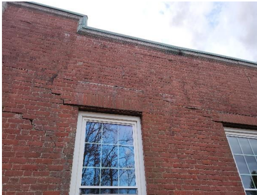
Typical East Wall Masonry Cracking
