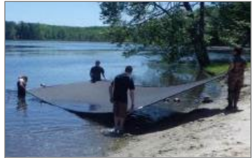
Benthic barrier installation
